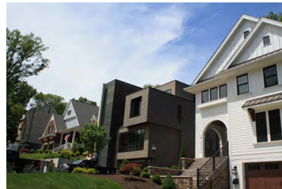
Four new single-family homes on Menlo Avenue
