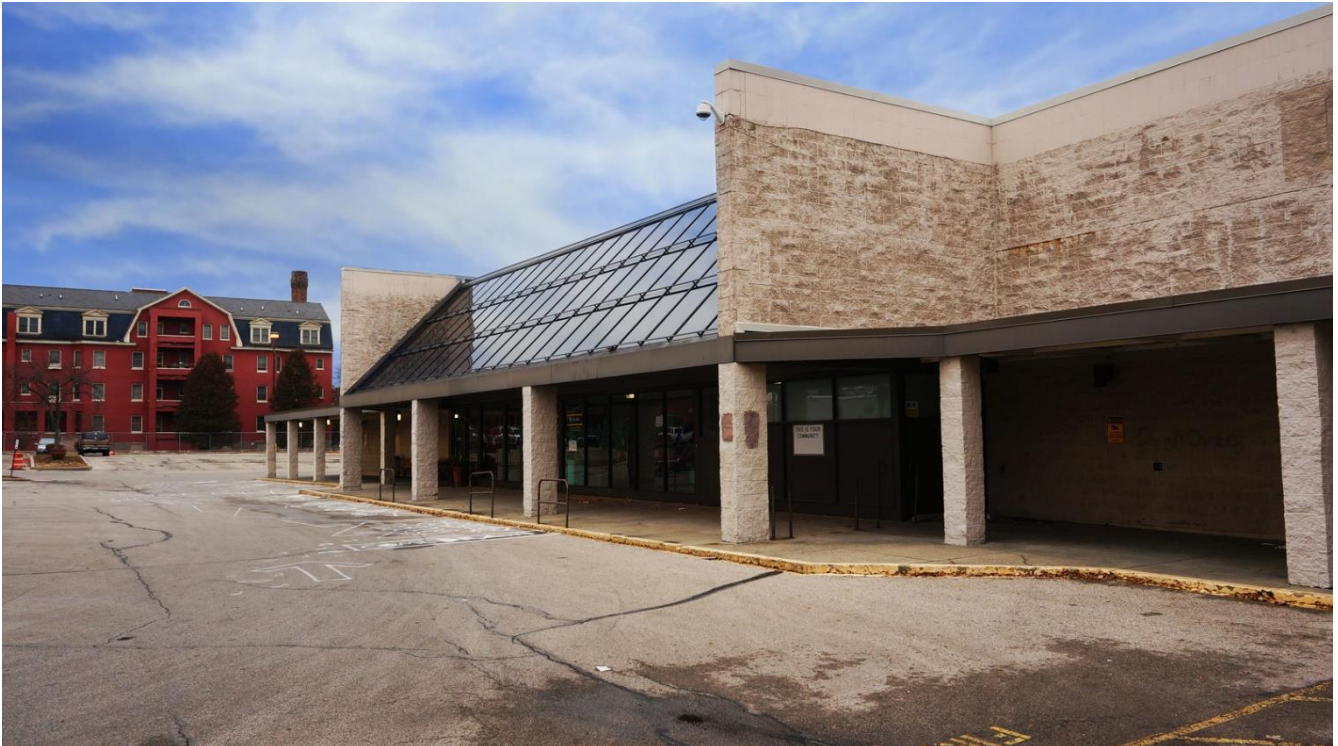
954 E McMillan – New Construction
