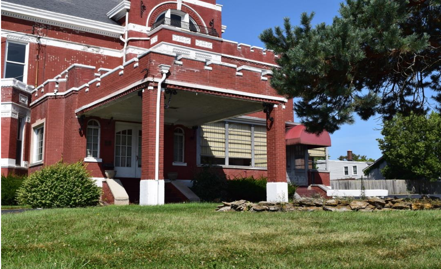
Detail of side addition
