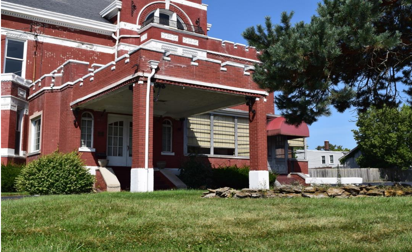
Detail of side addition
