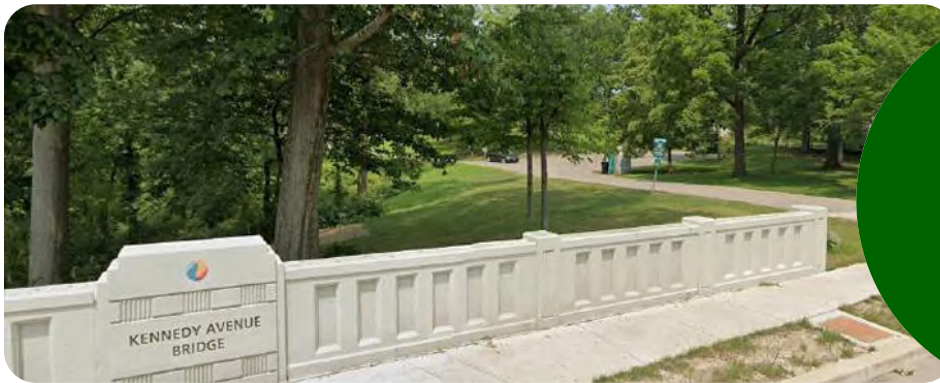
Kennedy Avenue Bridge & Kennedy Heights Park
