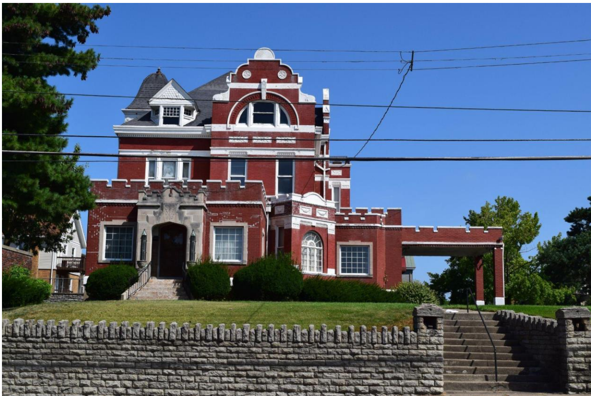
Figure 8: View of primary (south) facade, August 23, 2021.
