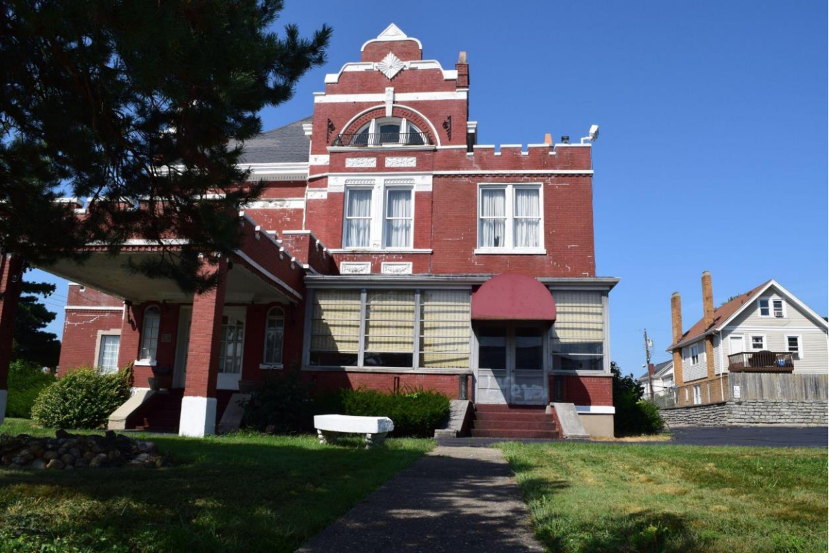
Figure 9: View of east elevation, August 23, 2021.
