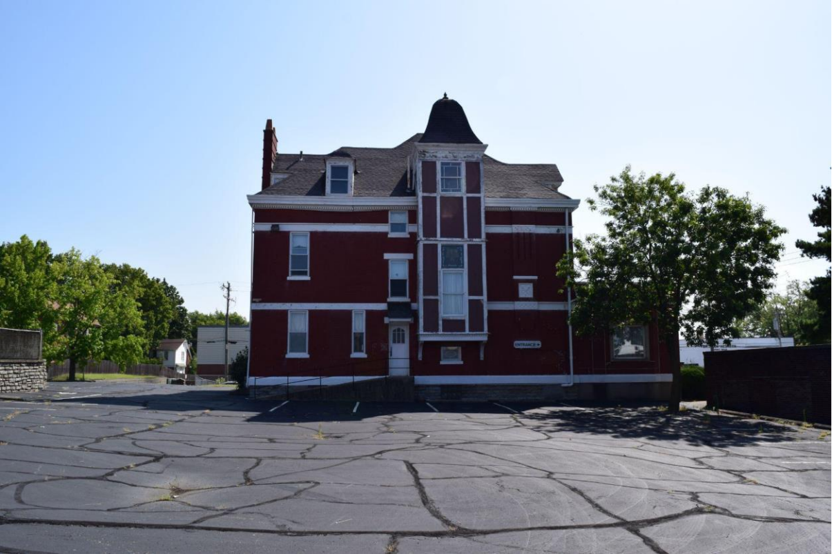
Photo 10: View of west elevation, August 28, 2021.
