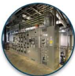
Battery Energy Storage
