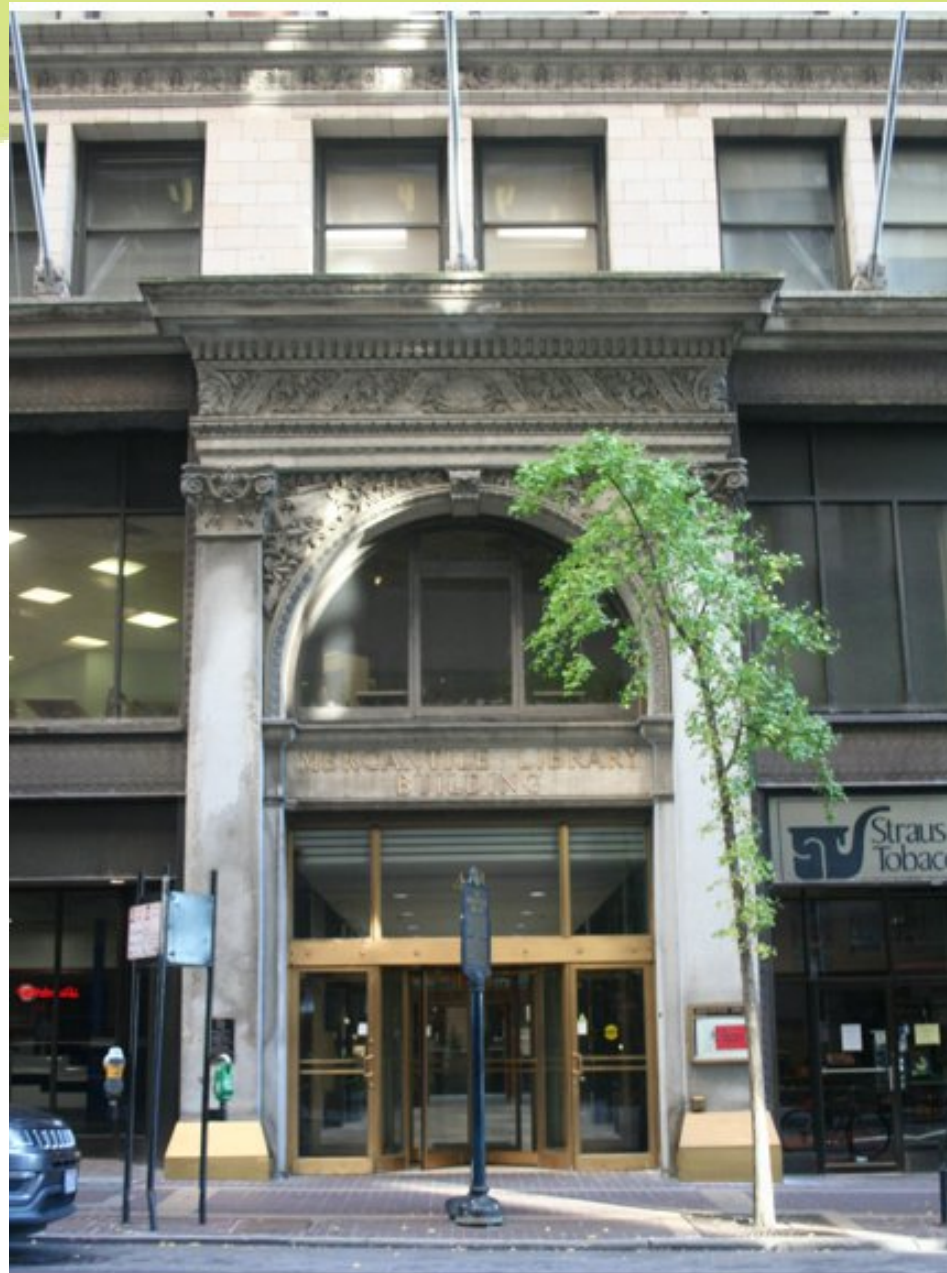
Mercantile Library Building, 414 Walnut Street, main entrance
