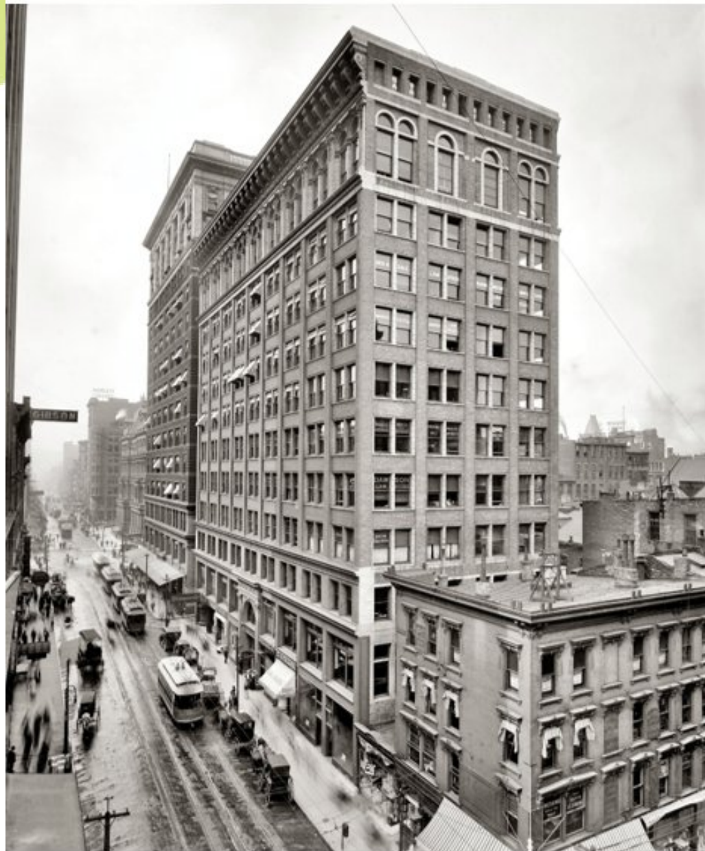
Figure 2. Historic photo of Mercantile Library Building, circa 1910, courtesy of The Mercantile Library
