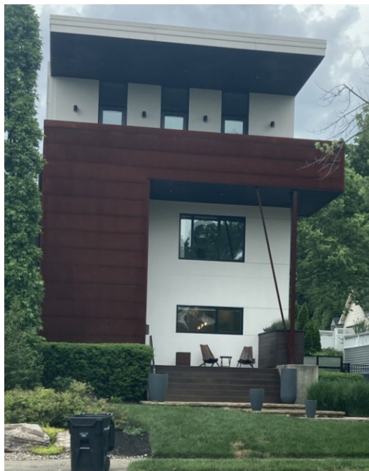
Figure 2 - Incompatible single family form 2872 Erie, could be re-configured as 3 family, 1 unit per floor.
