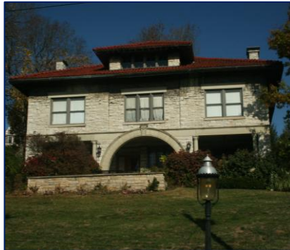
946 Redway Ave. (Elzner & Anderson)
