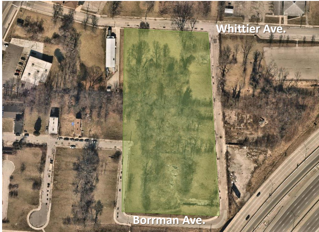
The Northeast Quadrant in the MLK and Reading Road Redevelopment Area of the Cincinnati Innovation District
