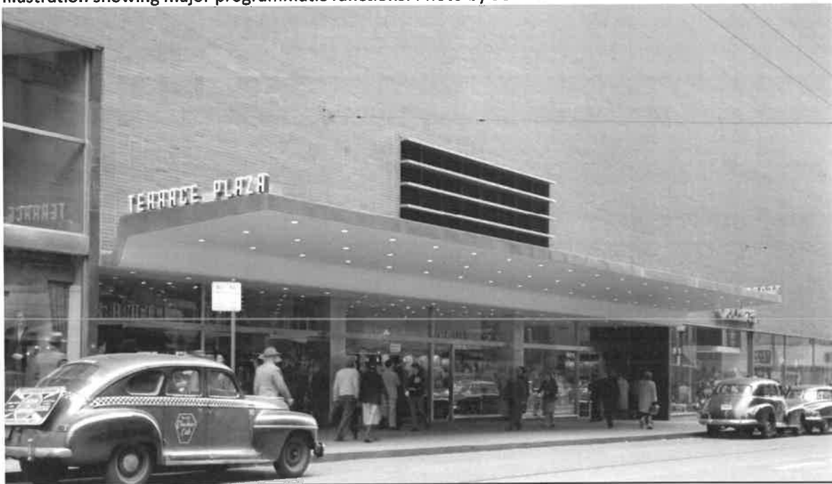
View of entrance, looking southwest, 1948, courtesy of Esto
