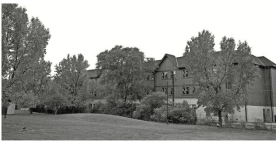
Developed by local nonprofits Over-the-Rhine Community Housing and Tender Mercies, the 62-unit Slater Hall was funded through the city's Affordable Housing Trust Fund. It sits behind a daycare and local recreation center.
