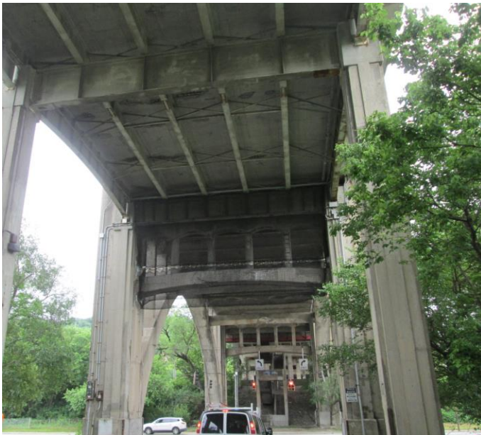
Debris netting under the Western Hills Viaduct west of Spring Grove Avenue
