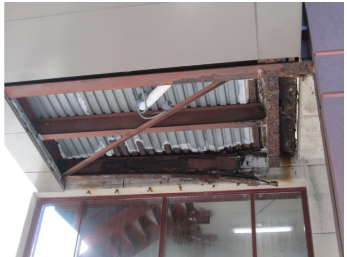
Above and below: Deteriorated floorbeam at the Plum Street Pedestrian Overpass north of 6 th Street.
