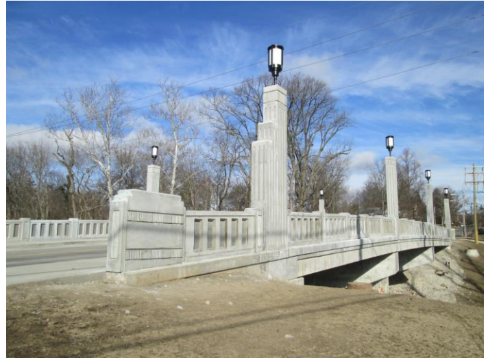
Kennedy Ave Bridge over IORY after reconstruction
