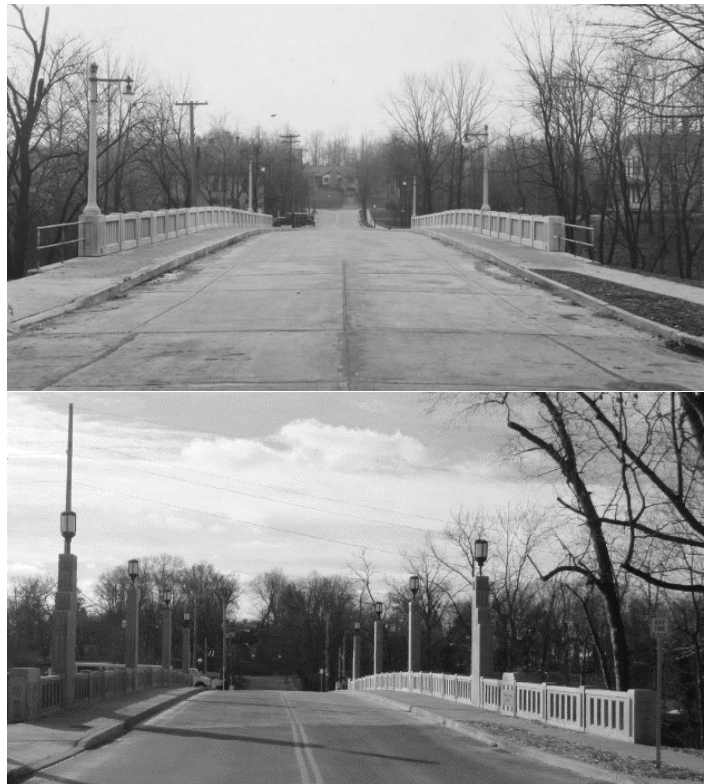
Kennedy Ave Bridge 1933 and 2020
