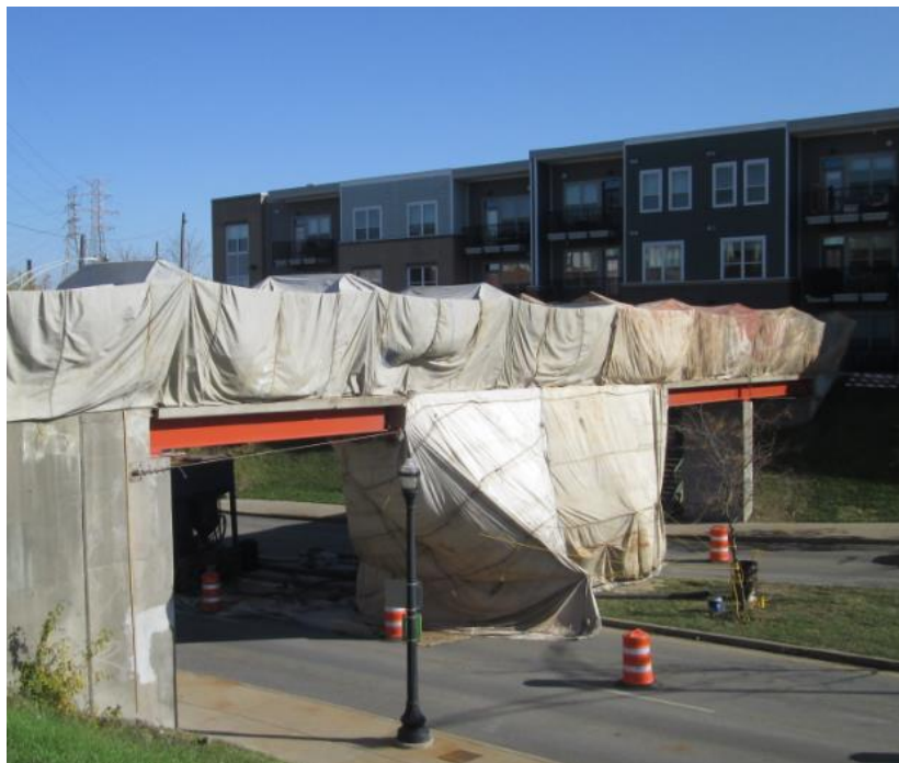
Bridge repair work at pedestrian bridge over Madison Rd in Oakley.
