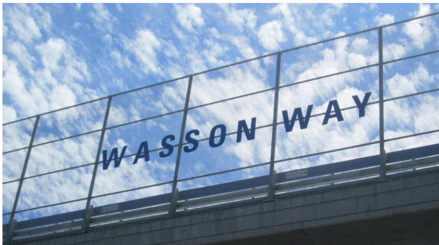
Newly installed Signage on the Wasson Way Bridge over I-71
