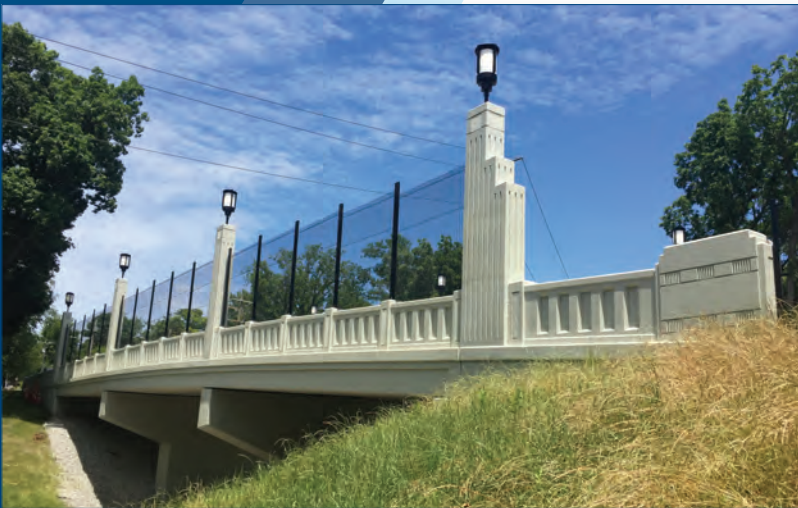
Kennedy Ave Bridge
