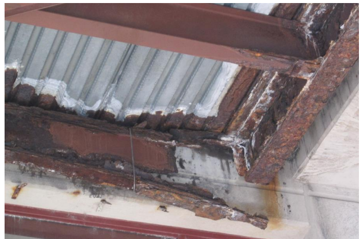
Above and below: Deteriorated floorbeam at the Plum Street Pedestrian Overpass north of 6 th Street.
