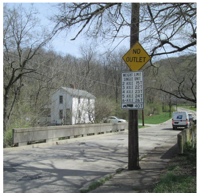
East Fork Bridge with Load Posting Sign
