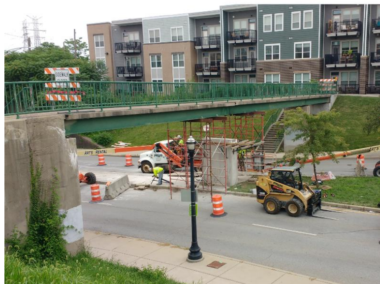
Construction activity at the Madison Road Pedestrian overpass west of IORY
