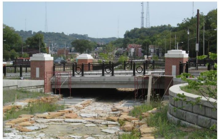
Above: Quebec Rd Bridge - Deck Area: 2,379 SF, SMF = 1
