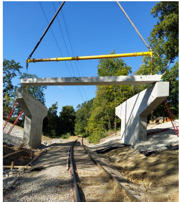
Setting the first beam of the Kennedy Ave Bridge over IORY
