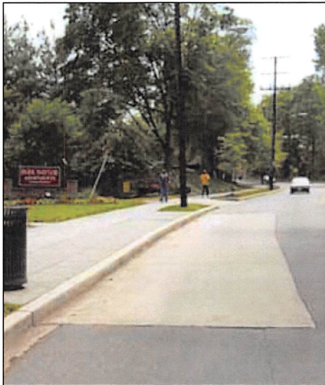
Figure 31: Example of Concrete Bus Pad
