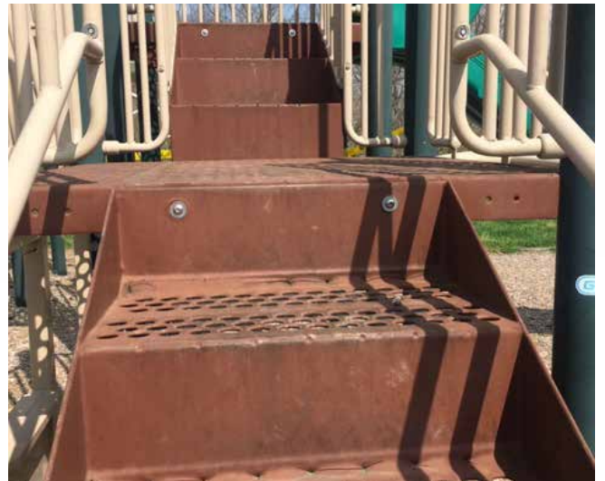
8. Maple Ridge worn play equipment
