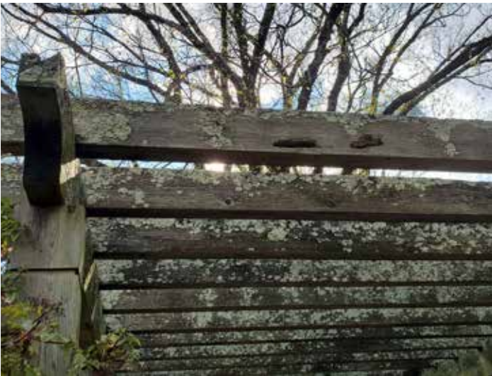
7. Lichens and insect damage at Ault Pergolas
