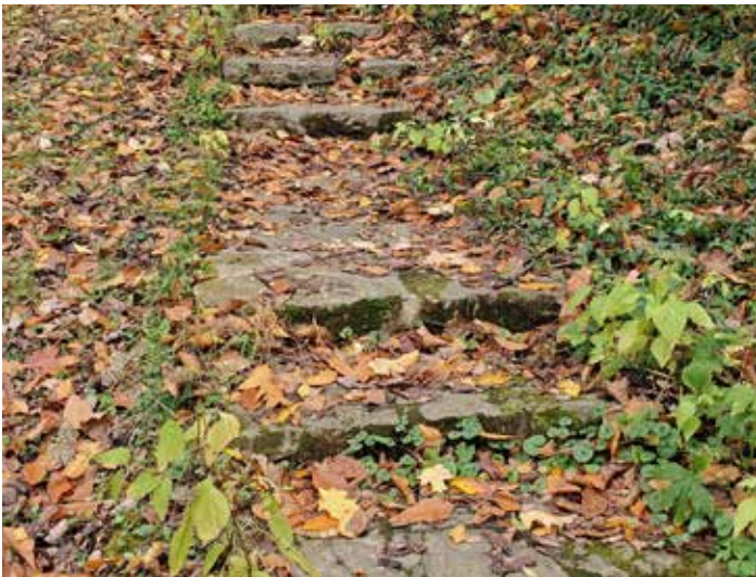
13. Kennedy Heights steps with no railing
