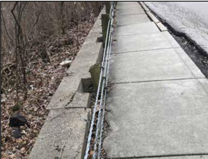
7. Wall, walk, and paving at Eden Park
