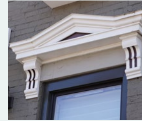
Decorative metal header at 1418 Elm Street.
