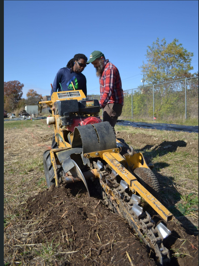
Anthony learns how to use a trencher in the building of an urban orchard
