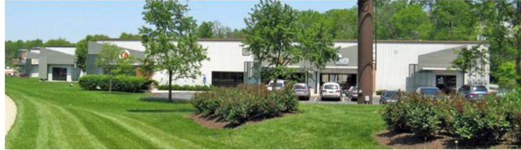
View from Red Bank Expressway and Red Bank Road, facing northward
