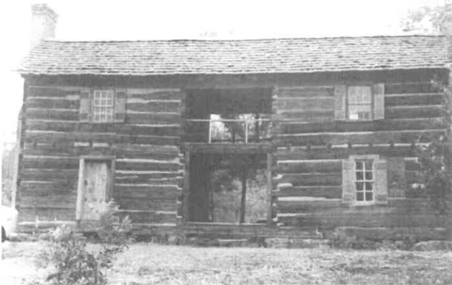
Looney House, Asheville vicinity, St. Clair County, Alabama. Examples of vernacular styles of architecture can qualify under Criterion C. Built ca. 1818, the Looney House is significant as possibly the State's oldest extant two-story dogtrot type of dwelling. The defining open center passage of the dogtrot was a regional building response to the southern climate. (Photo by Carolyn Scott).
