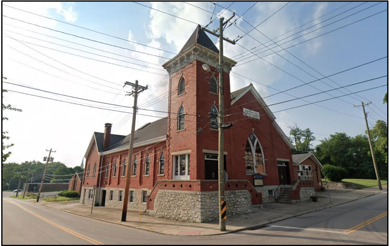
Figure 2. Image of subject property facing southeast ca. July 2022. Image from Google.
