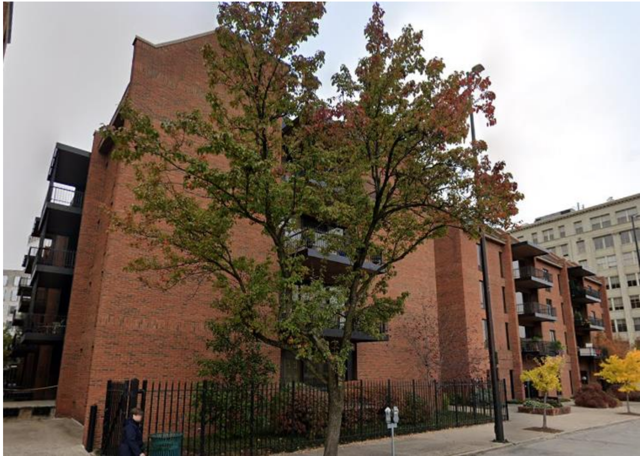
516 E. 4 th Street (aka 550 E. 4 th Street)
