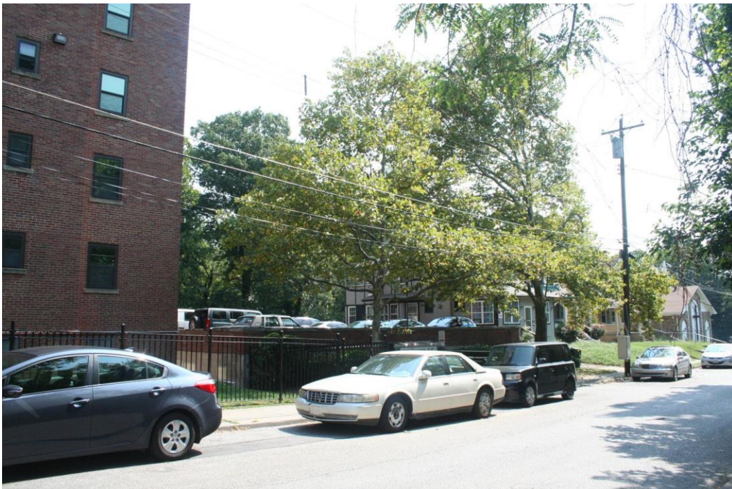
3700 Reading Road, view of parking garage to the east
