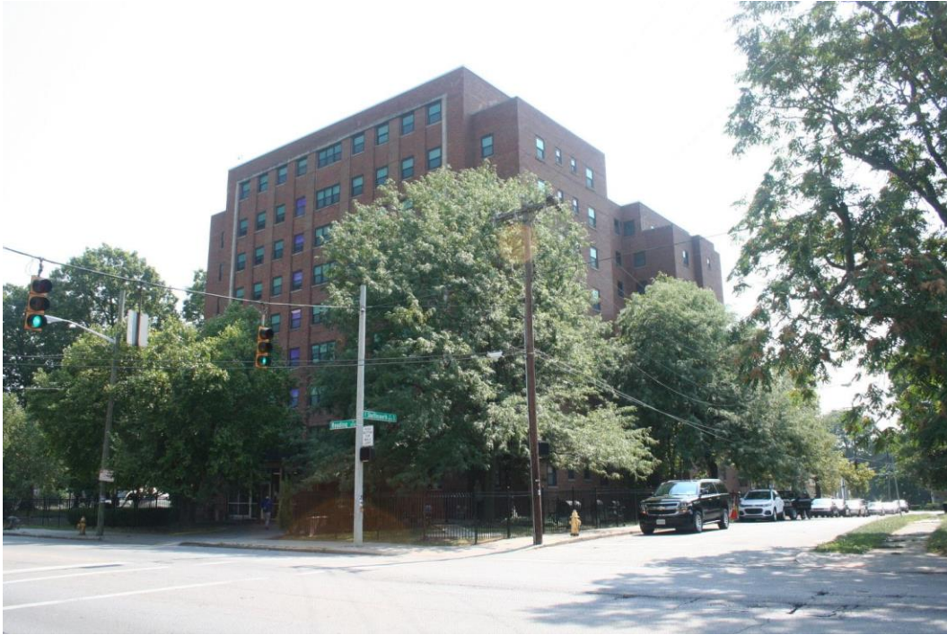
3700 Reading Road, Front (West) and South elevations
