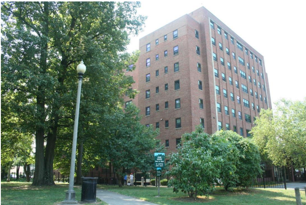
3700 Reading Road, North and East (Front) elevations
