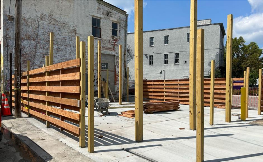
In Progress - 4024 Hamilton Ave
