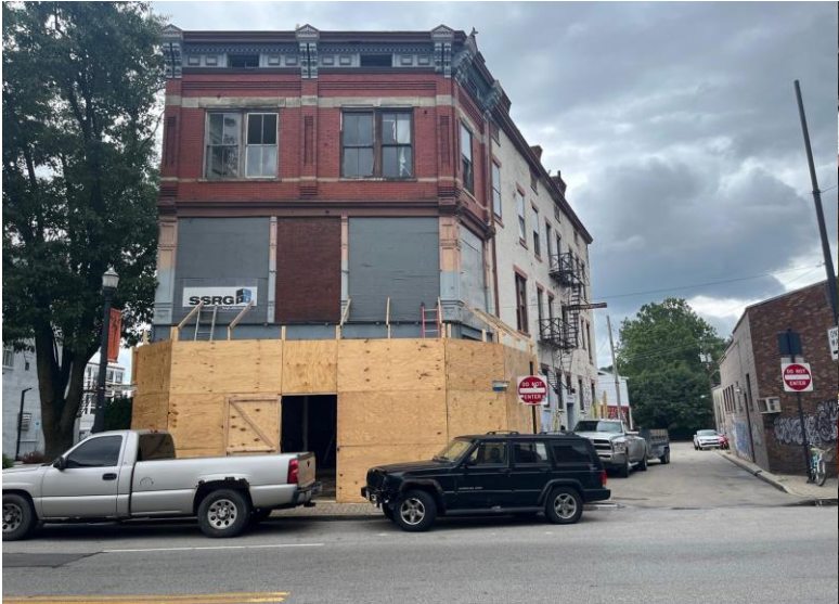
In Progress - 4024 Hamilton Avenue
