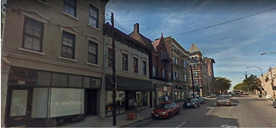
Before - Kemper Lane to Victory Parkway Streetscape
