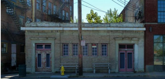
Before - Comfort Station Stabilization
