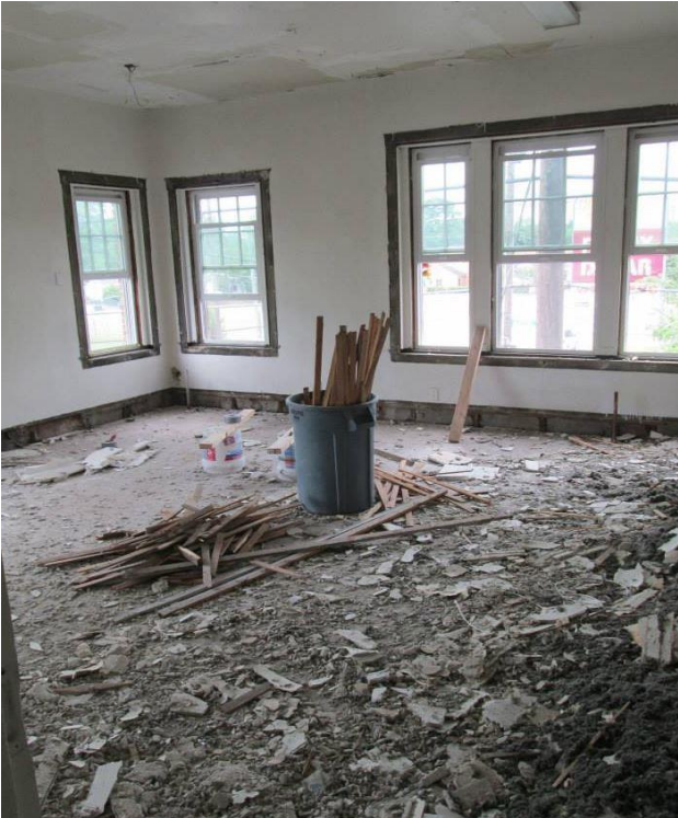
Before - Bank Building Kitchen
