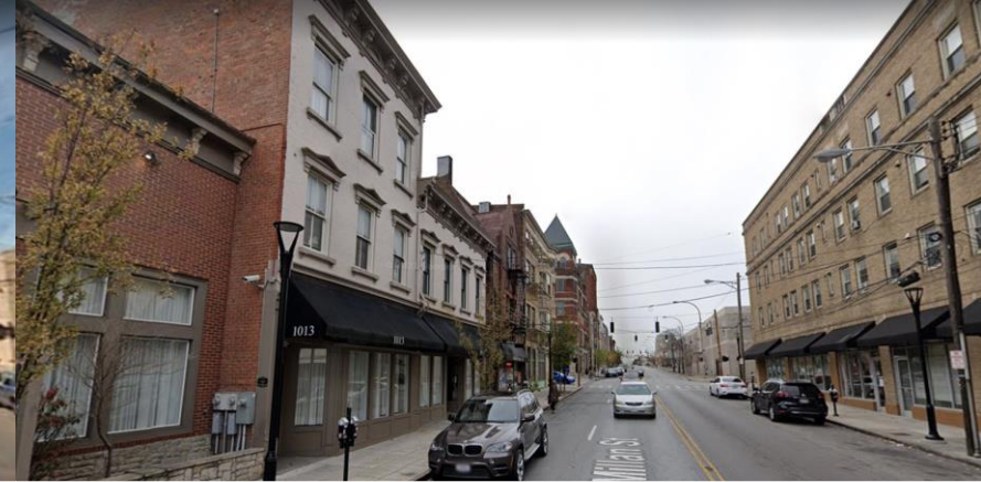
After - Kemper Lane to Victory Parkway Streetscape
