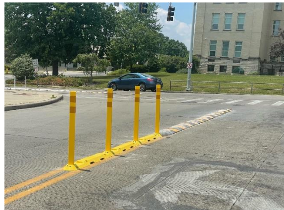
2 Clifton & Woolper Centerline Hardening (June 2023)
