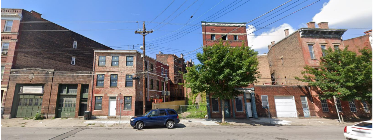
1804-1816 Vine Street, 29-31 E McMicken Avenue from E McMicken Avenue
