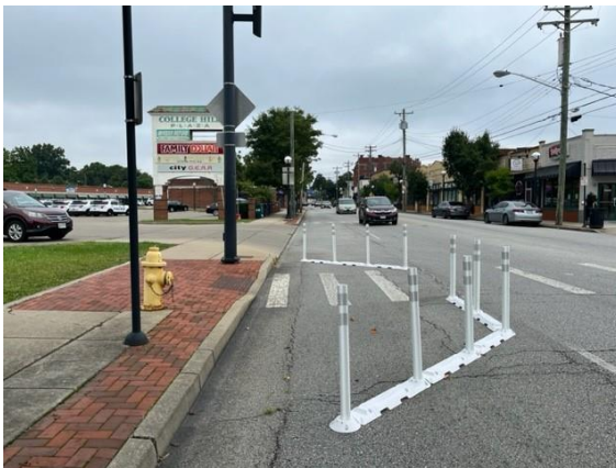
1 Hamilton Avenue quick curb bump-outs (August 2023)
