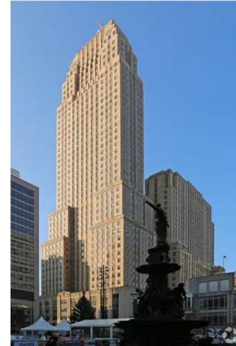
Carew Tower - Asbestos abatement for residential redevelopment in the Central Business District
