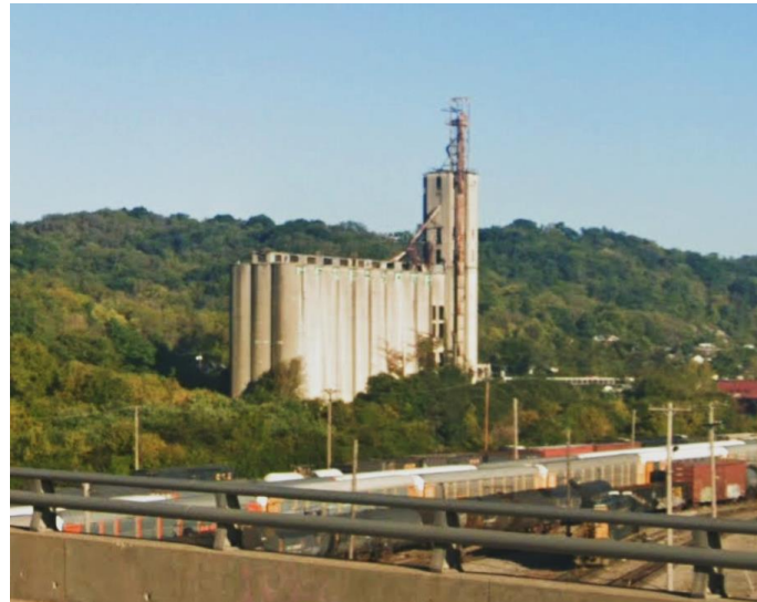
Grain Silos – Millvale
