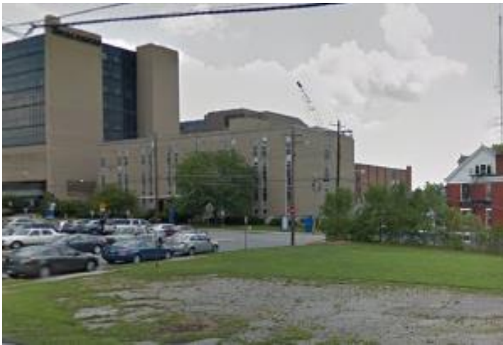
2605 University Court southeast view
