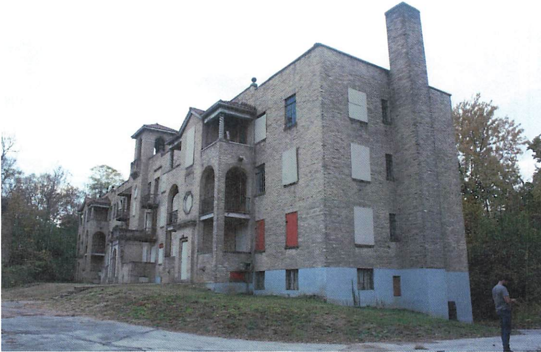
La Ventura, East (Front) and North (Side) Elevations
