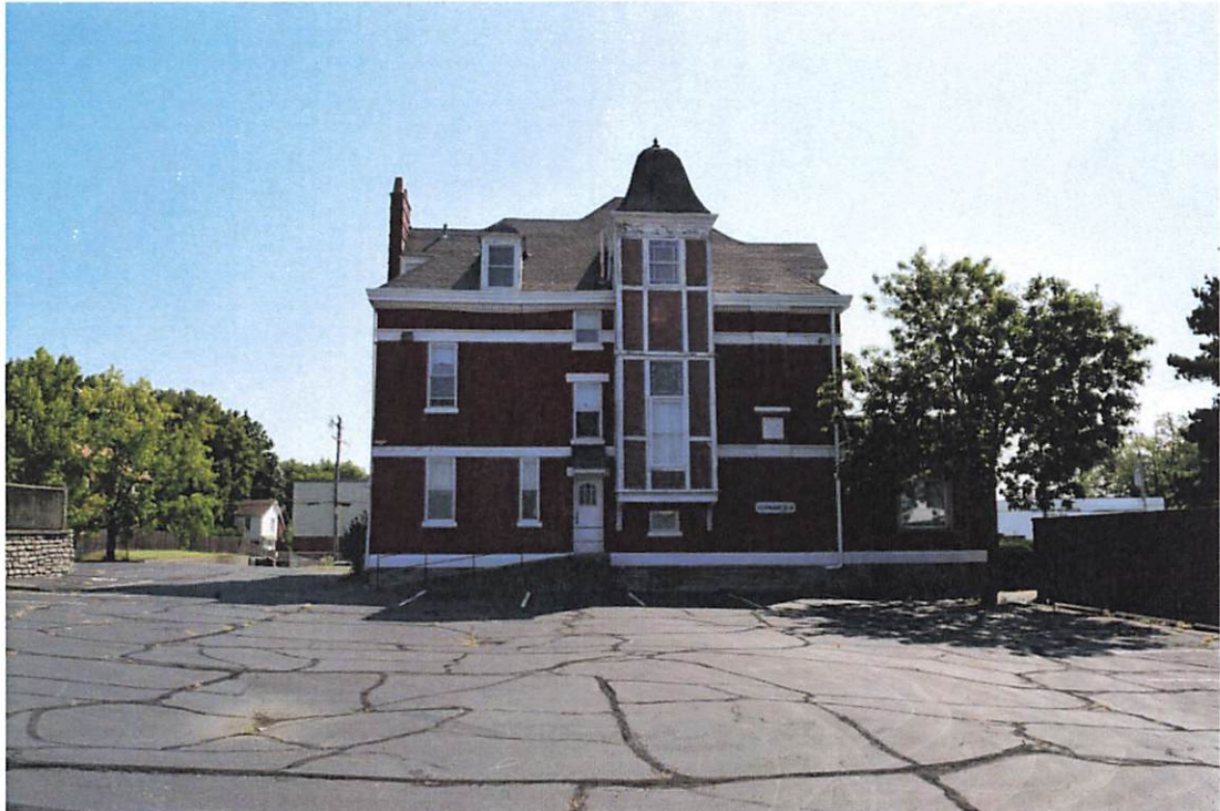
Photo 10: View of west elevation, August 28, 2021.
