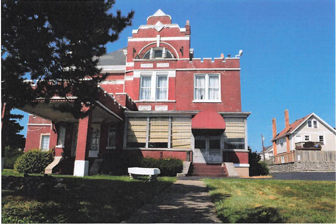
Figure 9: View of east elevation, August 23, 2021.
