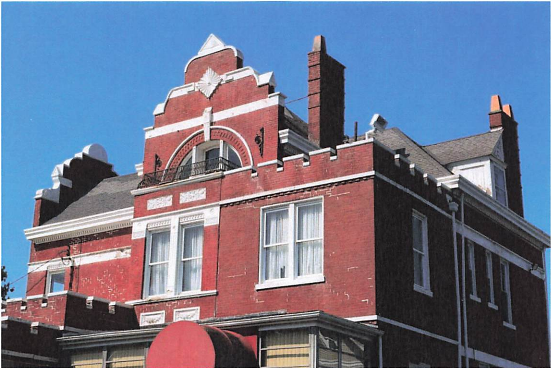
Photo 12: Detail of Second Story and Flemish parapeted gables, August 28, 2021.
