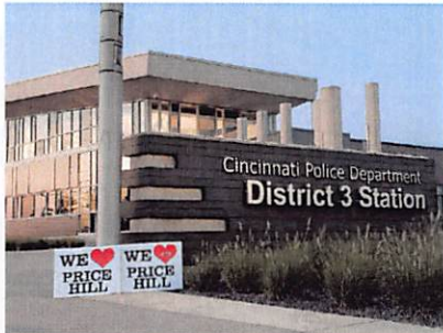
The Cincinnati District 3 Police Headquarters in Net Zero—producing all of the energy it needs to operate. Photo courtesy of Pete Witte.
