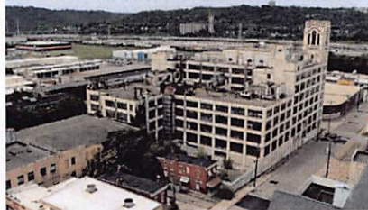
Historic Crosley building, a brownfield site in Camp Washington. Photo courtesy of Maddy Schmidt/WCPO.
