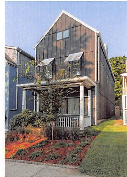
The upgrades to this historic Northside home demonstrate how existing buildings can help address the climate crisis. Photo courtesy of Casey Moothart.
