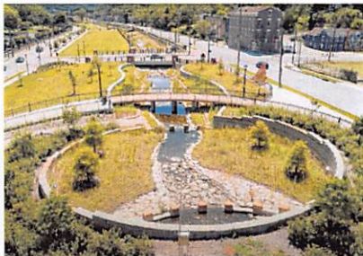
Lick Run Greenway, Green Infrastructure Project, Greater Cincinnati Metropolitan Sewer District. Photo courtesy of MSD.
