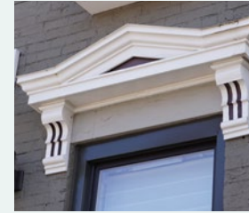
Decorative metal header at 1418 Elm Street.
