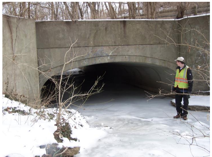
Berkshire Lane Culvert: Deck Area: 1767 SF, SMF = 1
