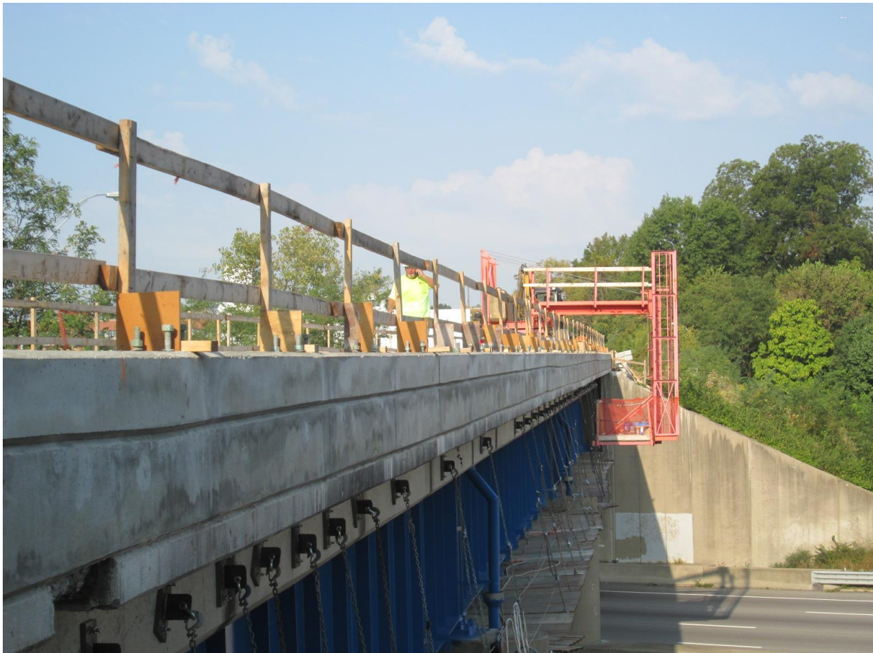
Wasson Way Bridge over I-71 - Rehabilitation
