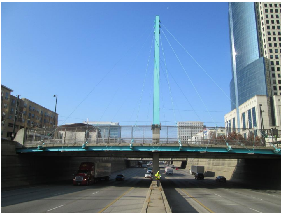
Routine Inspection of the bridges over Fort Washington Way
