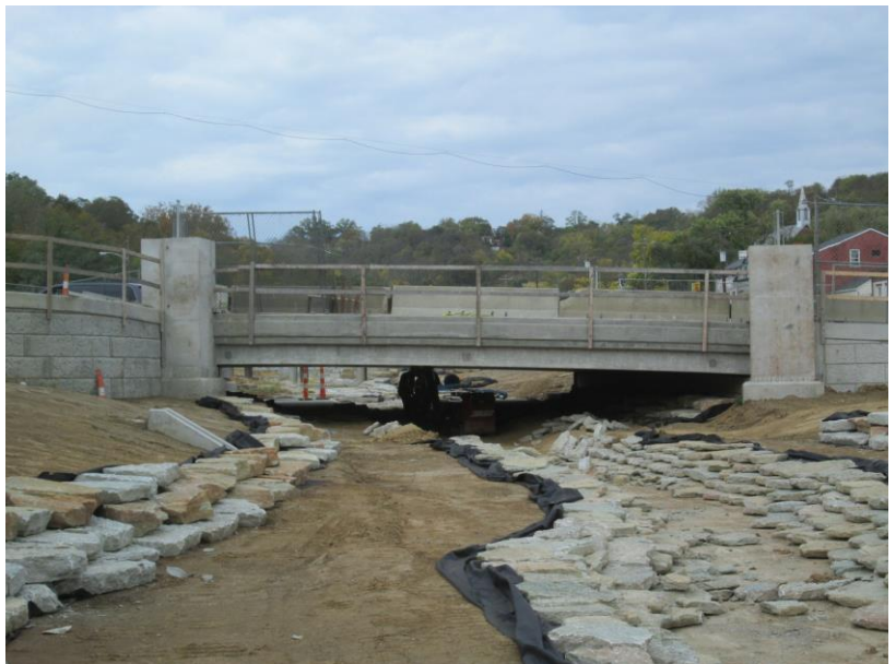
Van Hart Street Bridge over Lick Run
