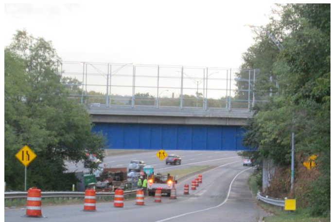
Wasson Way over I-71 during rehabilitation
