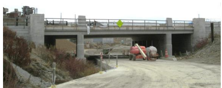
Construction of the Harrison Ave Bridge over Lick Run
