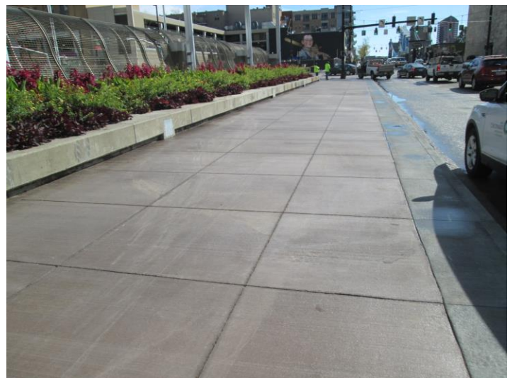
2019 Sidewalk Paver Replacement with colored concrete, Walnut Street Bridge over Fort Washington Way.
