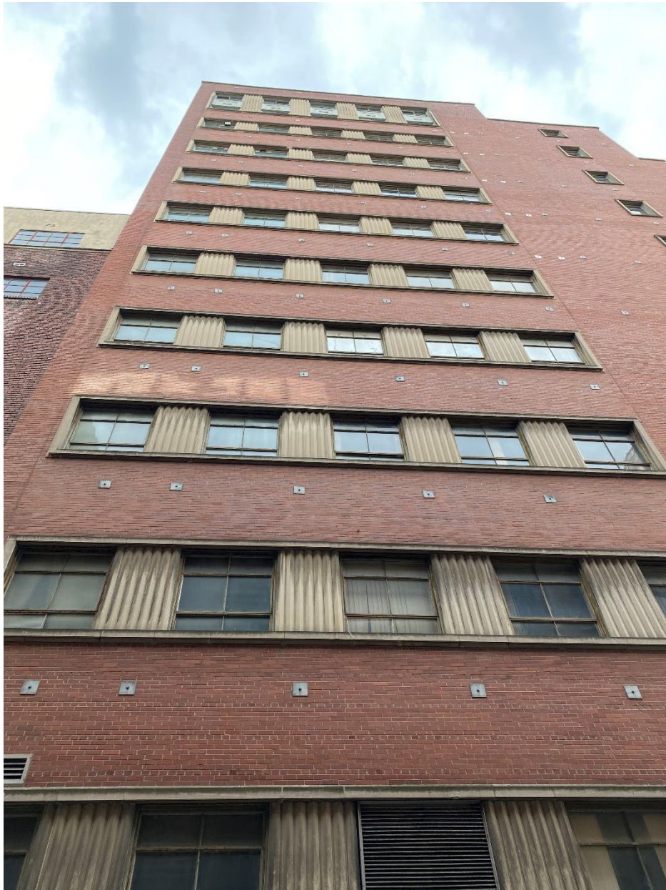
Photograph 11: North elevation looking west.
