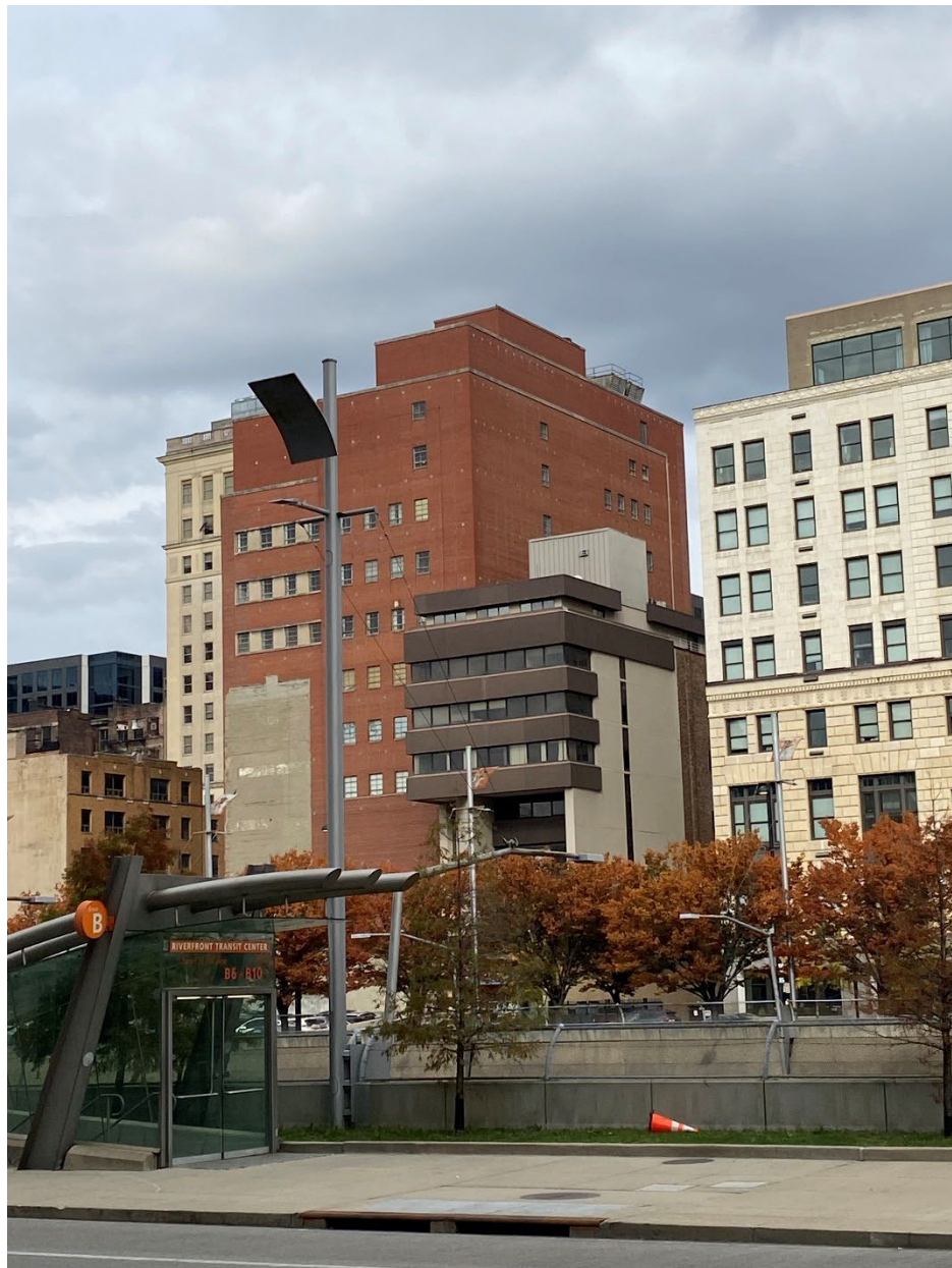
Photograph 9: South and east elevations looking northwest.
