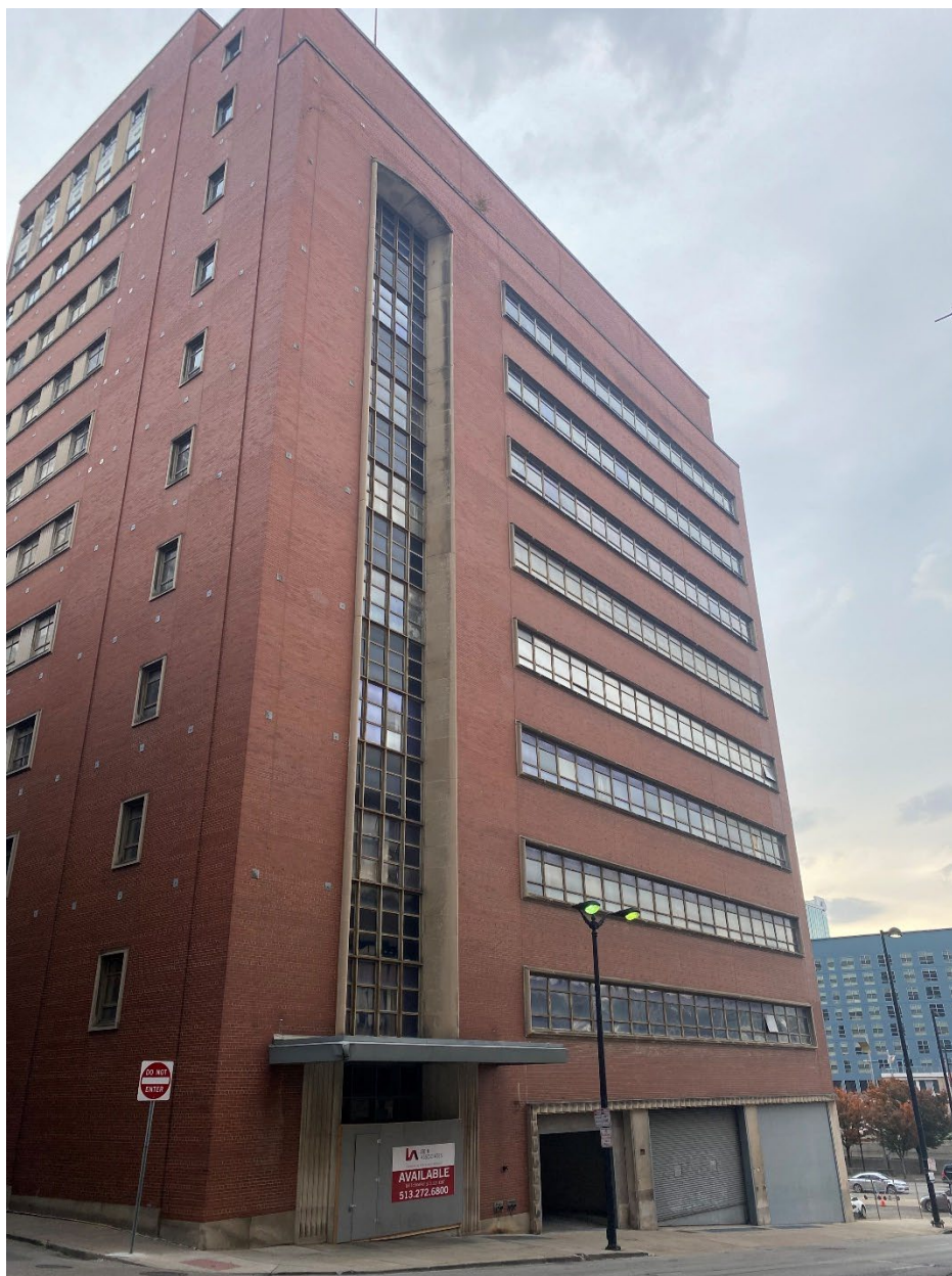
Photograph 2: Primary west elevation looking southeast.
