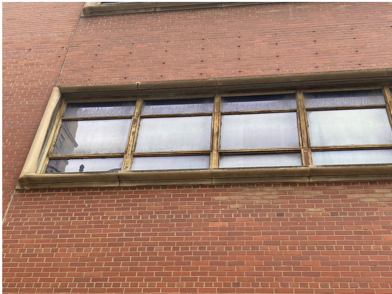
Photograph 7: West elevation looking east at second floor windows.
