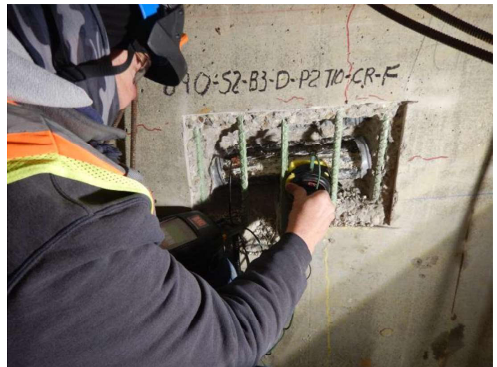
Above: PT investigation at 2 nd Street.
