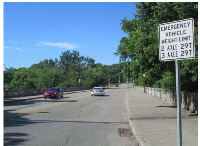
Above: Park Avenue Bridge over Kemper Lane with Load Posting sign for Emergency Vehicles.
