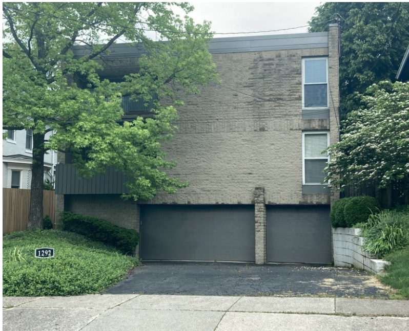
Figure 3 - Incompatible multi-family box at 1292 Michigan
