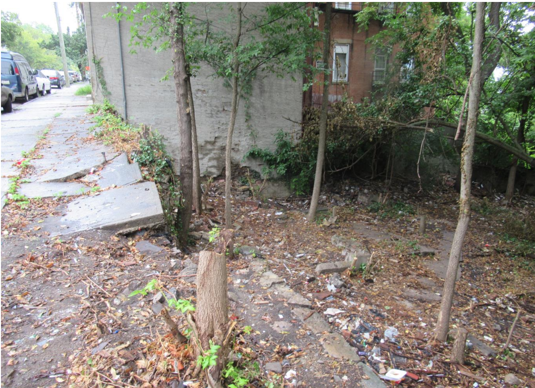
2550-54 BEEKMAN ST -CLEANED JULY 28, 2021
