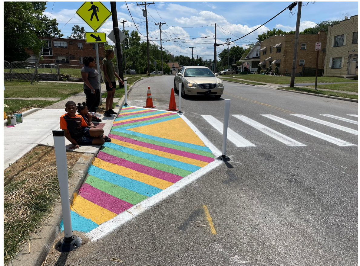
Painted curb extension on McHenry Ave in East Westwood
