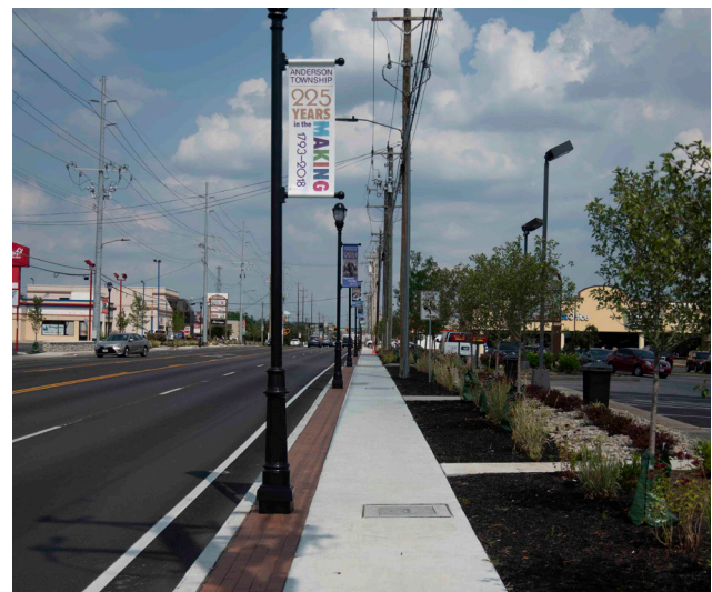
Example of the buffer between vehicles and pedestrians
