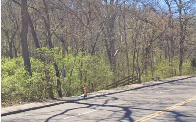
Current sidewalk conditions between Virginia Avenue and Highforest Lane along Colerain Avenue
