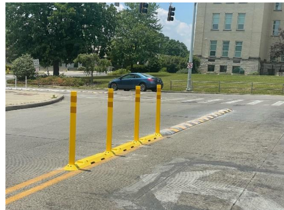
2 Clifton & Woolper Centerline Hardening (June 2023)
