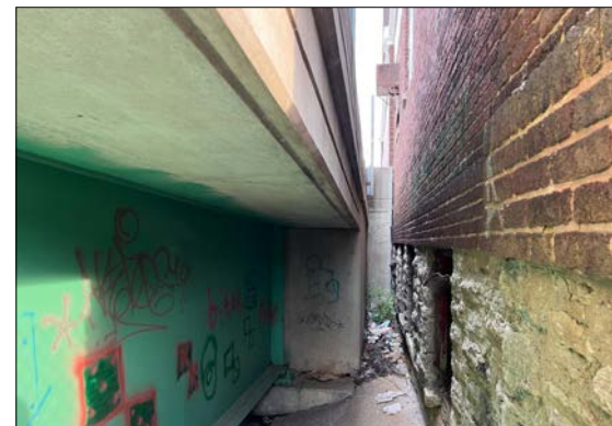
8 VIEW OF EXISTING BUILDING ADJACENT TO LUDLOW VIADUCT
