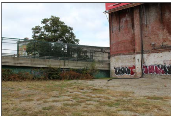
7 VIEW OF EXISTING BUILDING ADJACENT TO LUDLOW VIADUCT
