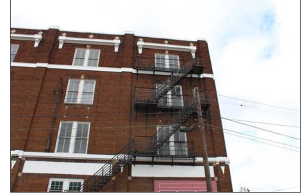
3 VIEW OF EXISTING FIRE ESCAPE
