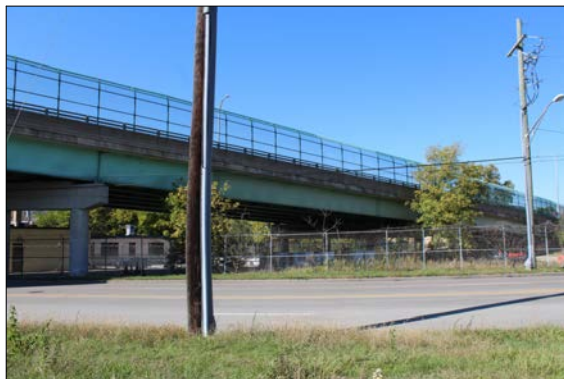
4 VIEW OF LUDLOW VIADUCT FROM WILLAM DOOLEY BYPASS
