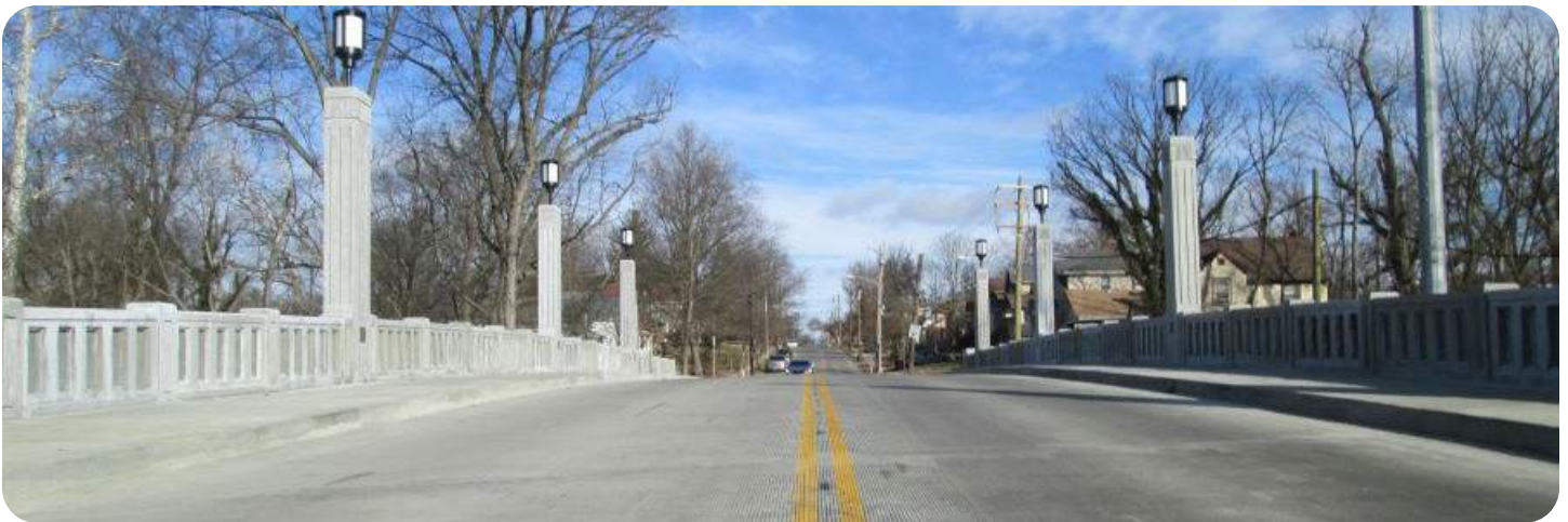
Kennedy Avenue bridge between Woodford Road and Northdale Place opened in 2020 Source: City of Cincinnati DOTE
