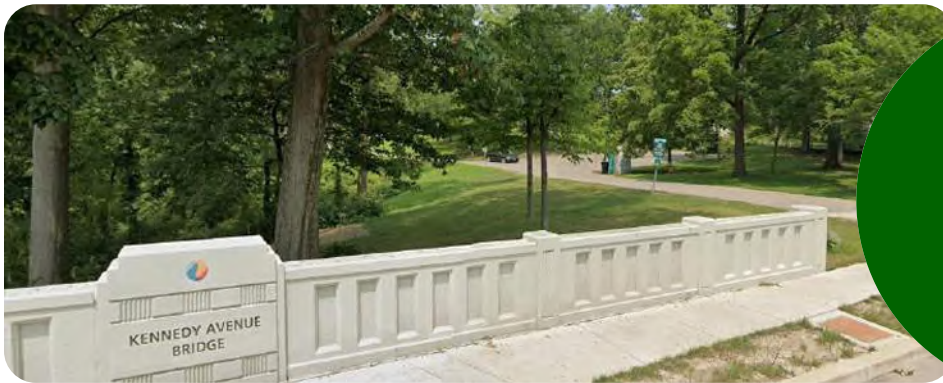
Kennedy Avenue Bridge & Kennedy Heights Park
