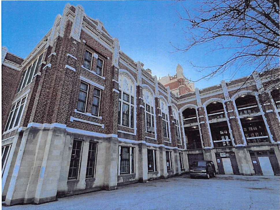
Rear elevations of the school
