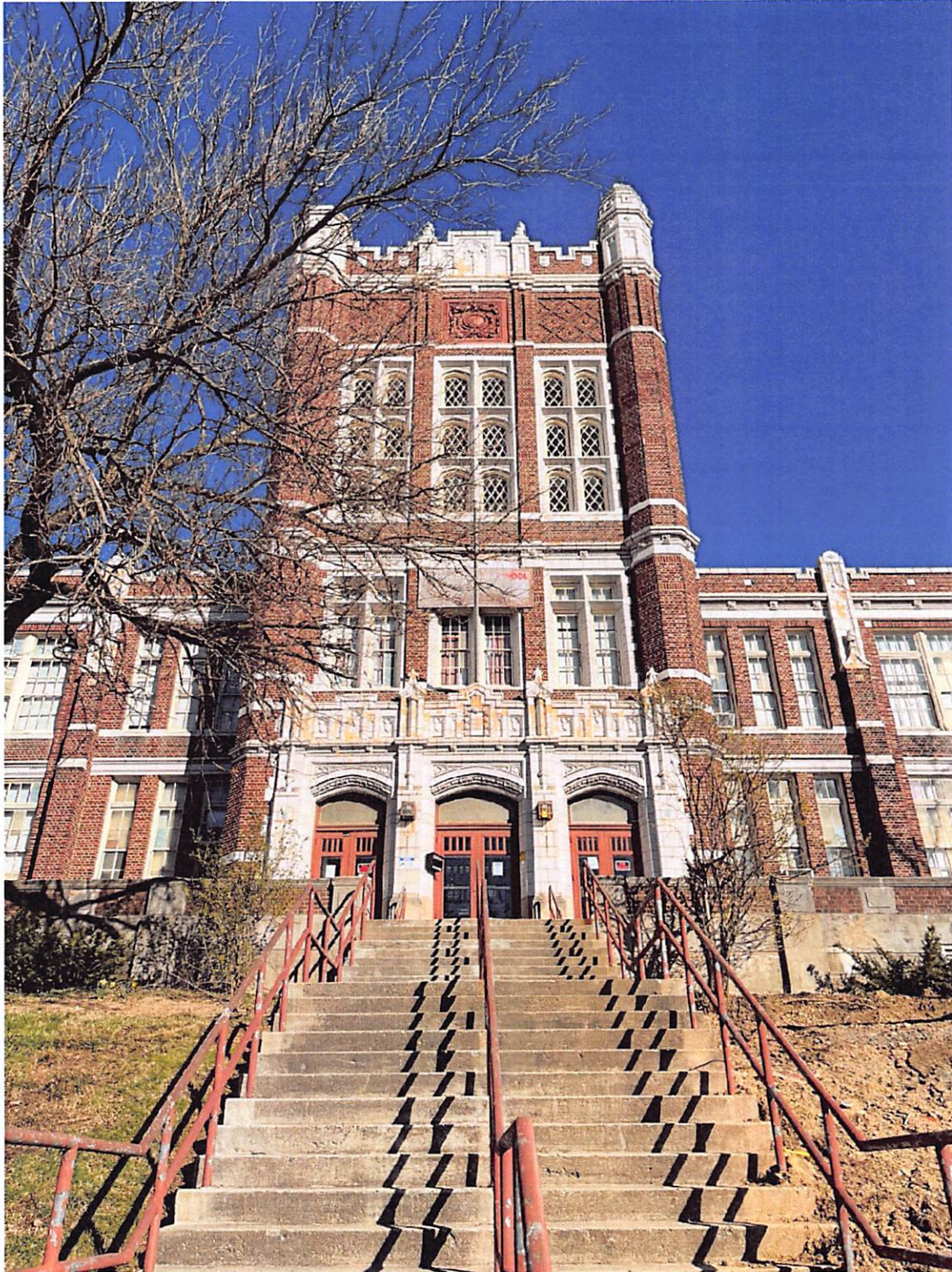
Front Entrance of the school and tower
