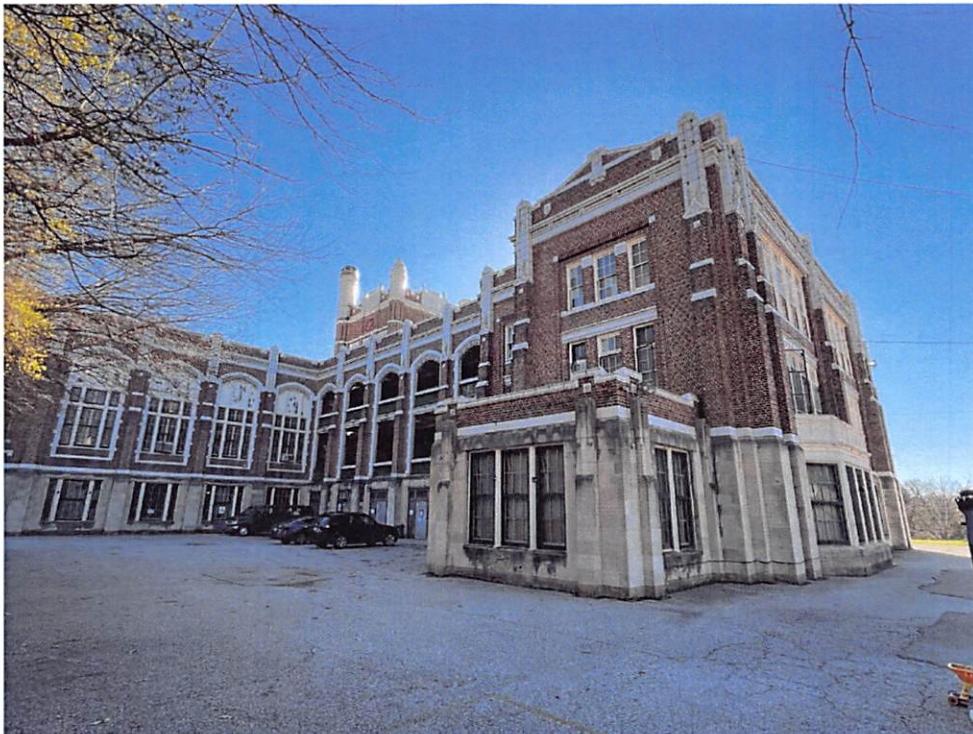
North and rear elevations of the school
