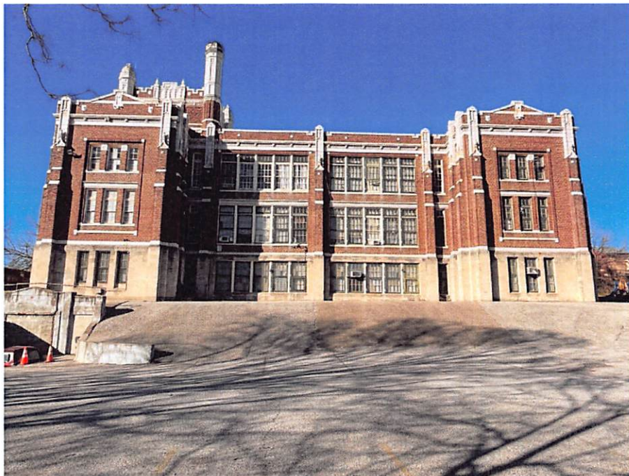
South elevation of the school
