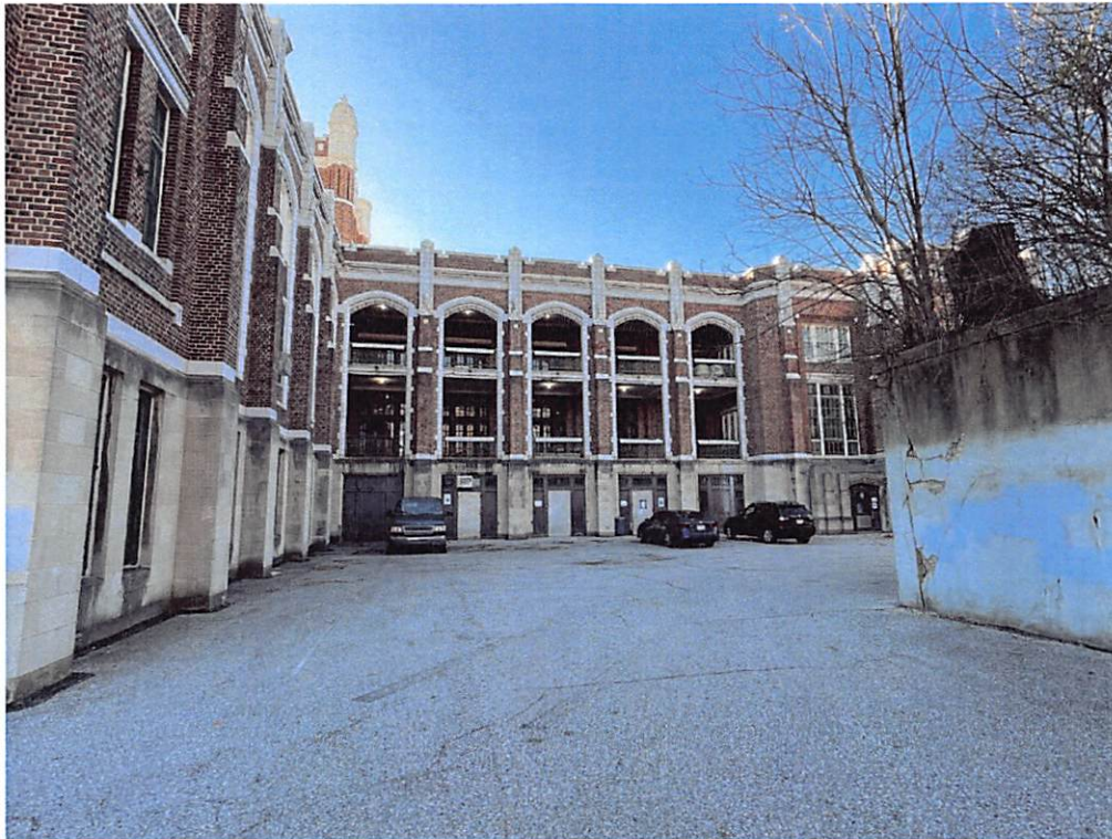
South elevation of the school
