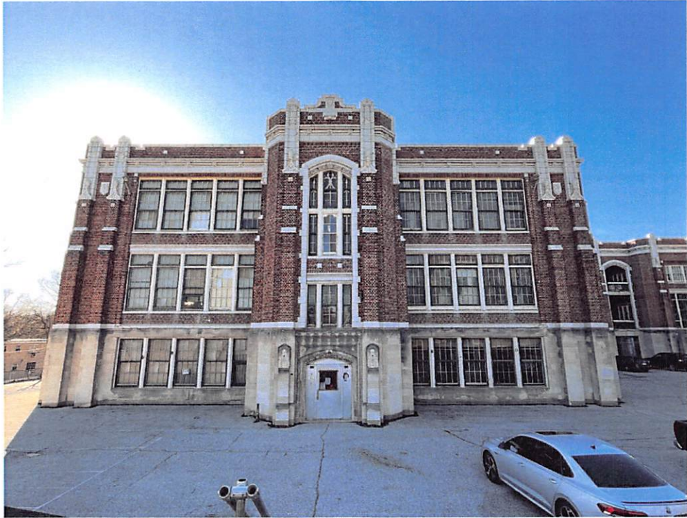
South elevation of the school
