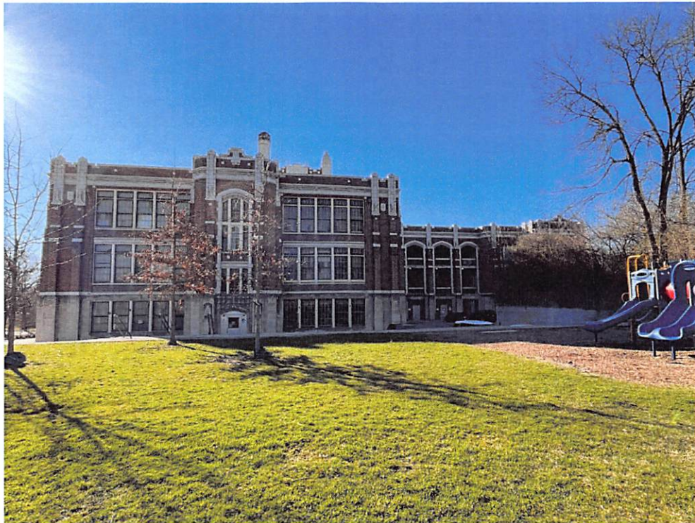
South elevation of the school
