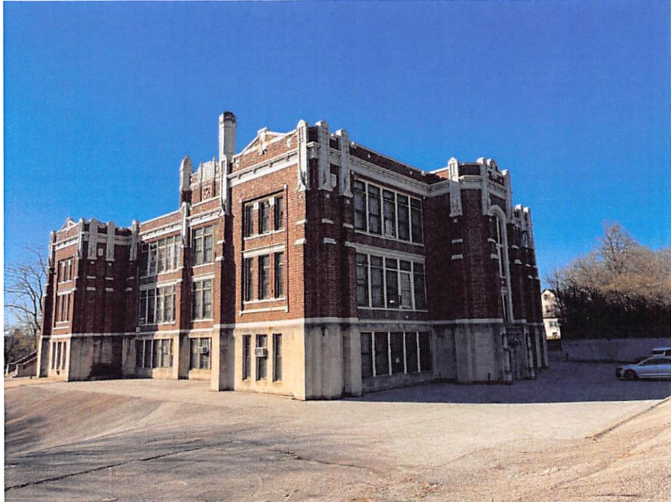
South side and rear of the school
