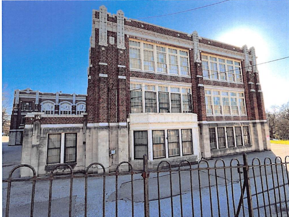
East elevation of the school
