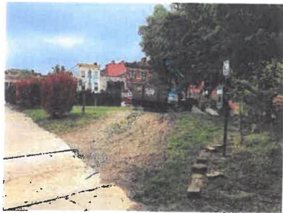
2600 Short Vine Street – Corry Street View
