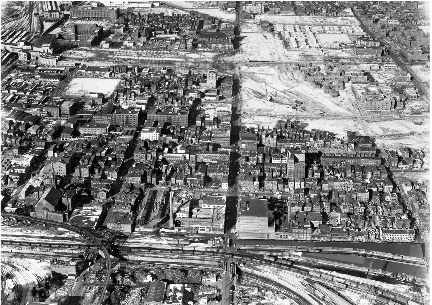
Demolition of Lower West End for Interstate 75. Photo from jjakucyk.com
