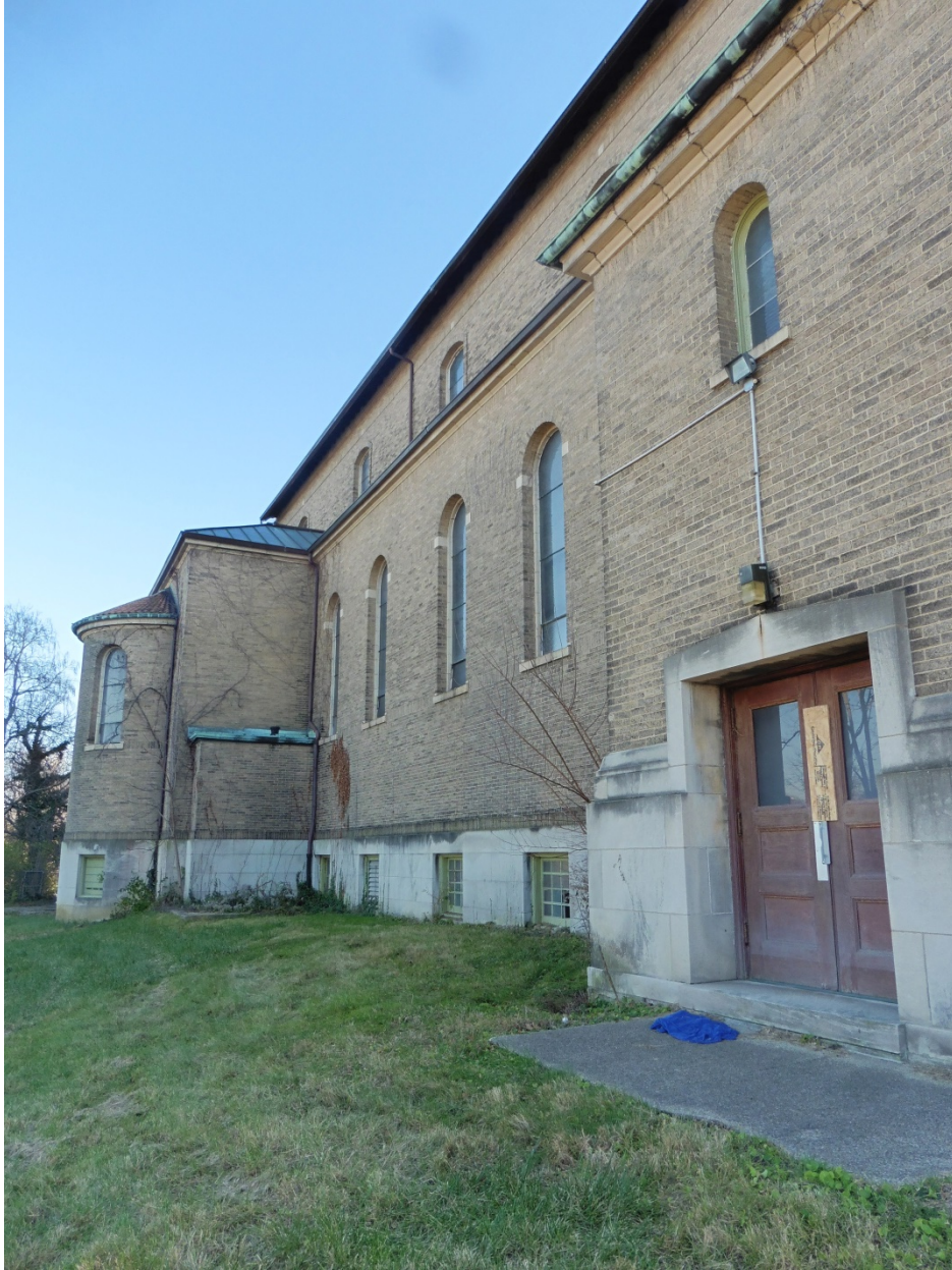
Figure 4 View of north elevation of church building, from the southeast.
