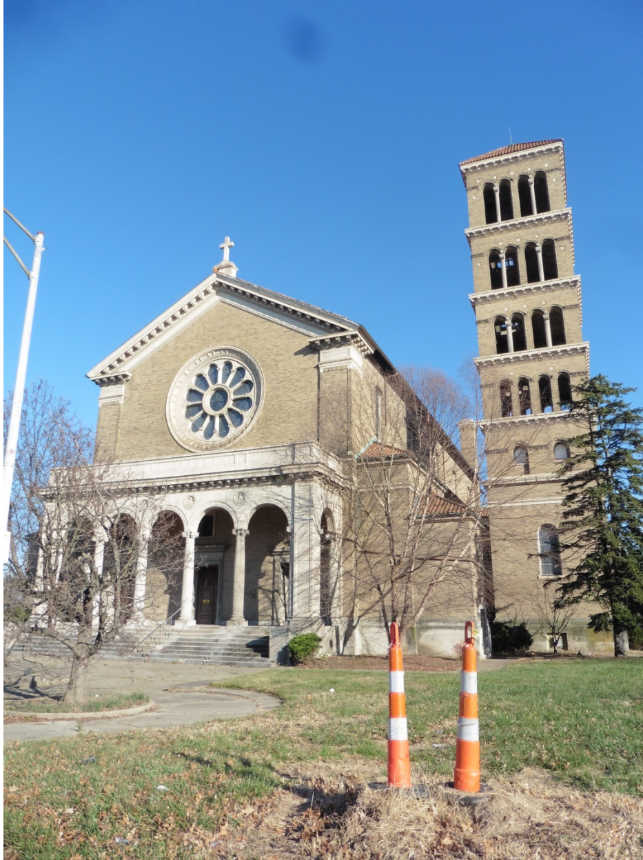
Figure 3 Close-in view of church and campanile from front lawn. View to the NE.
