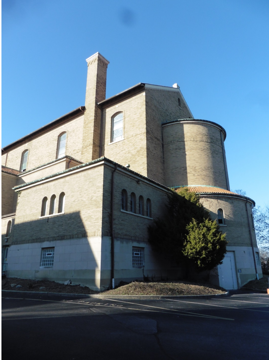
Figure 5 Partial view of rear facade, with semicircular apse, and south elevation. View to the NW.
