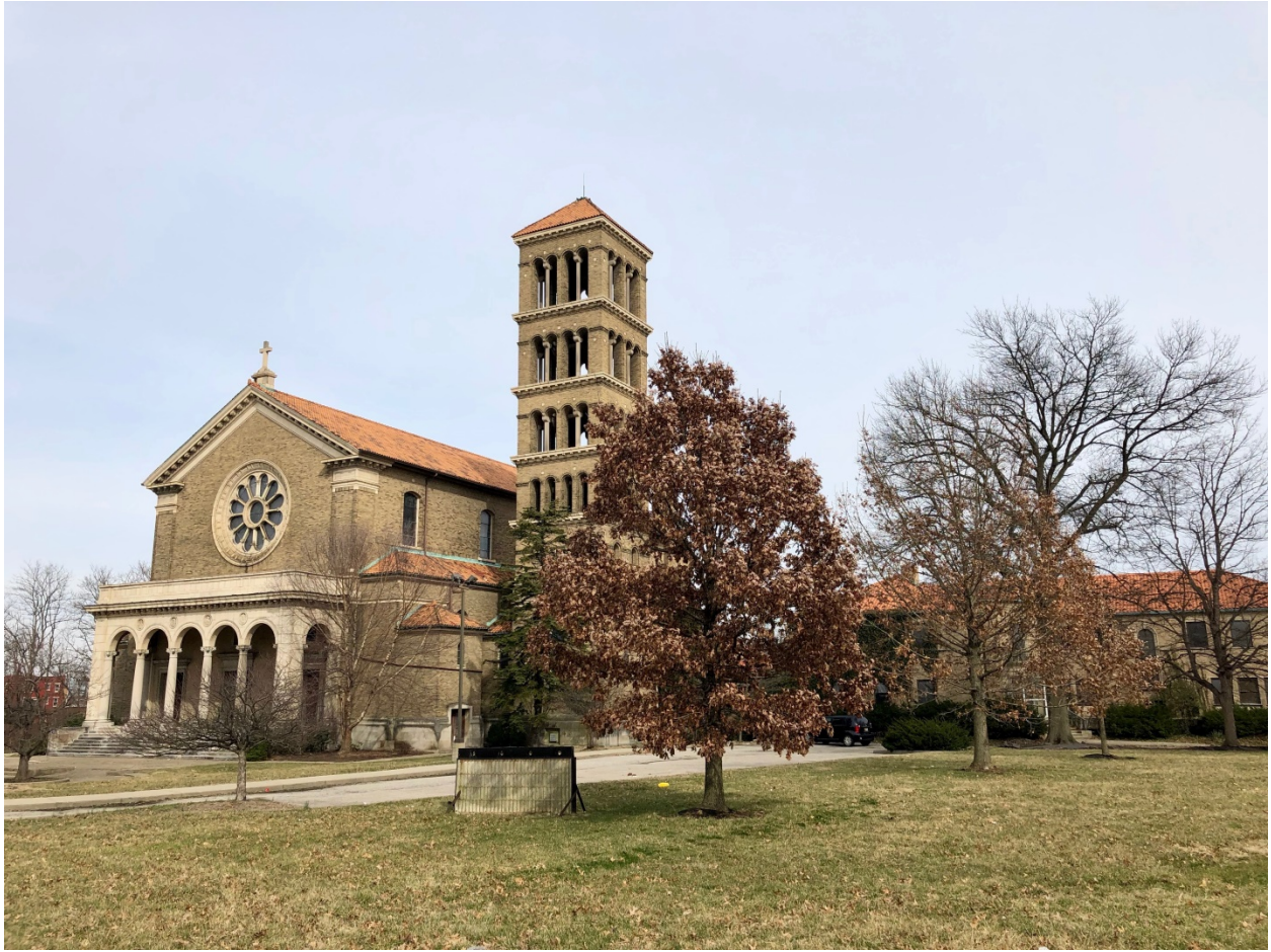
Figure 1 Overall view of St. Mark's Church from Montgomery Road. View to the NE.
