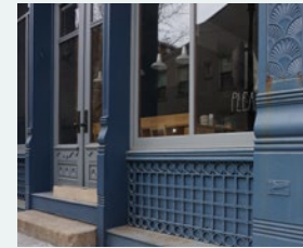
Decorative cast iron storefront at 116 East 14th Street.
