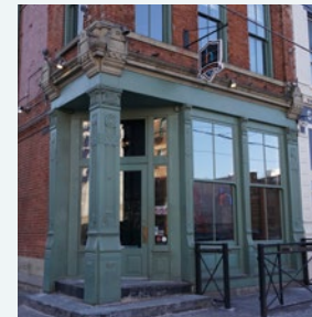
119 E 12th Street exhibits the characteristics of commercial storefronts.
