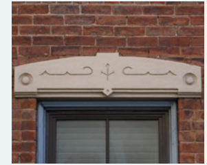
Decorative stone lintel at 1431 Elm Street.
