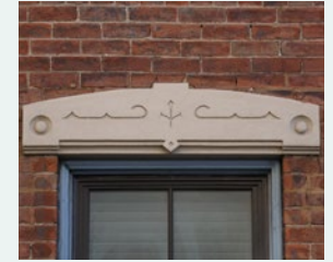
Decorative stone lintel at 1431 Elm Street.
