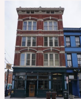
1126 Walnut exhibits the characteristics of grouped window openings.
