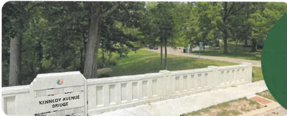
Kennedy Avenue Bridge & Kennedy Heights Park
