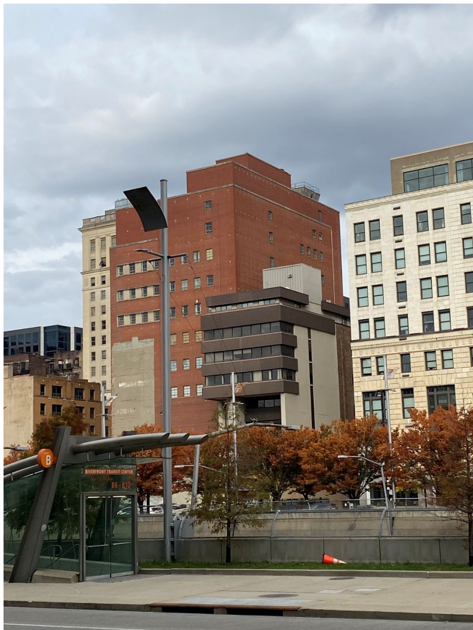
Photograph 9: South and east elevations looking northwest.
