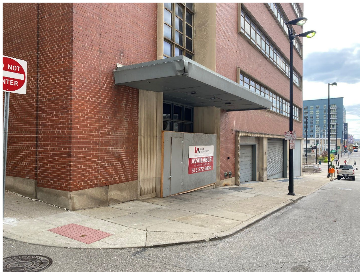
Photograph 5: West elevation looking southeast at entrance.
