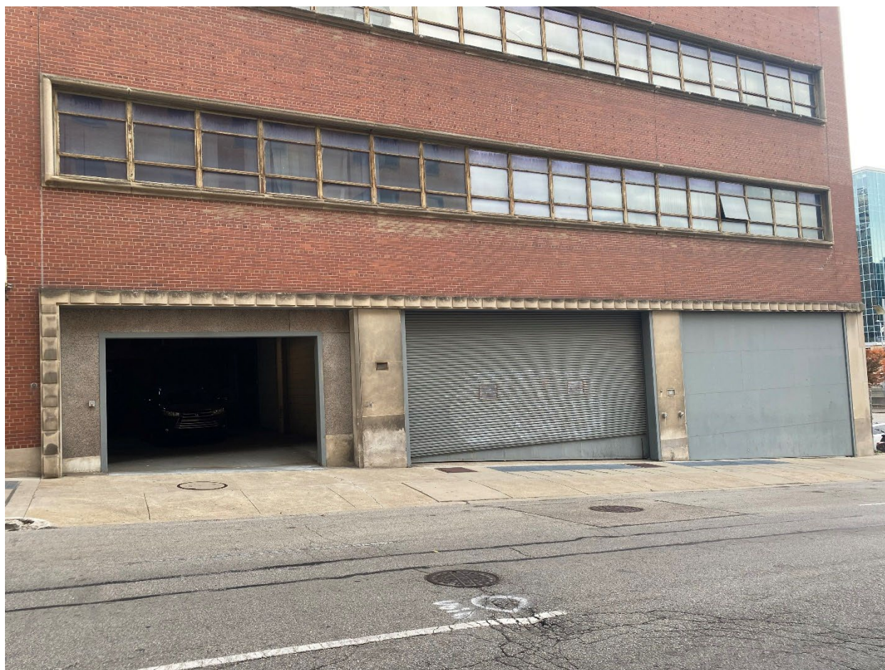
Photograph 6: West elevation looking east at loading bays.
