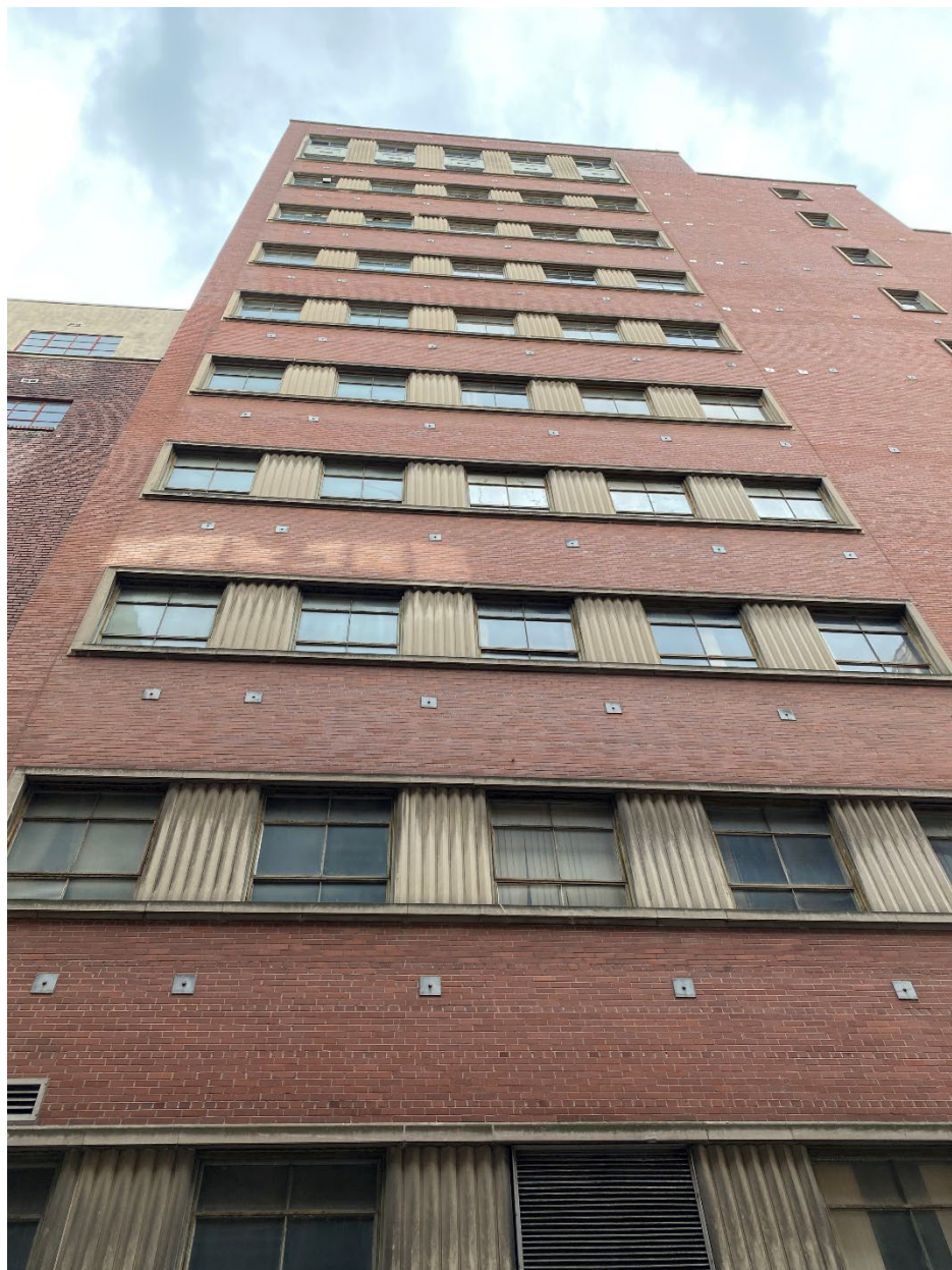
Photograph 11: North elevation looking west.
