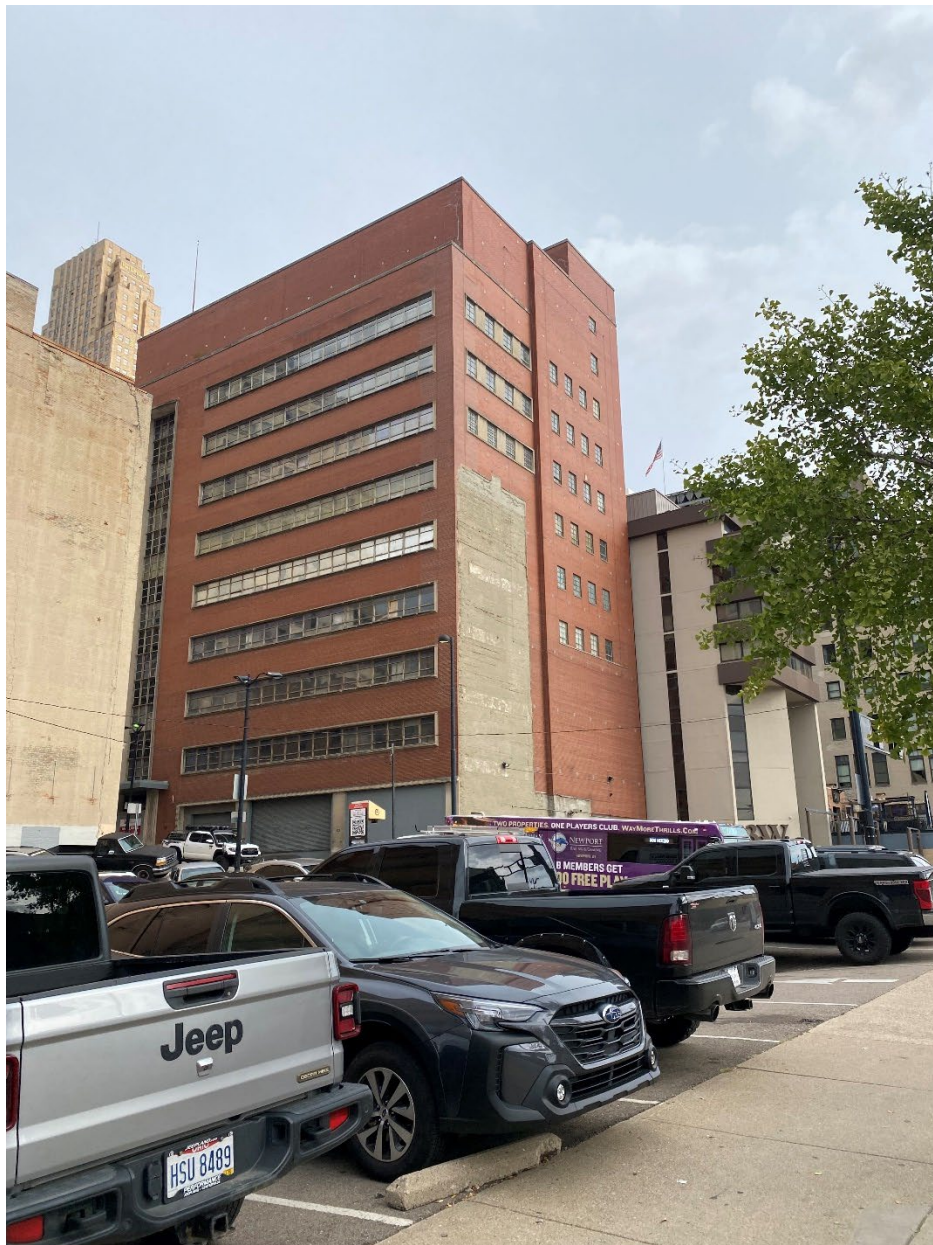
Photograph 3: West and south elevations looking northeast.
