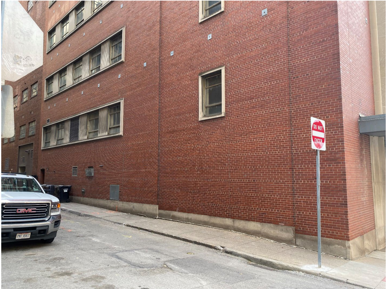
Photograph 10: North elevation looking southwest.
