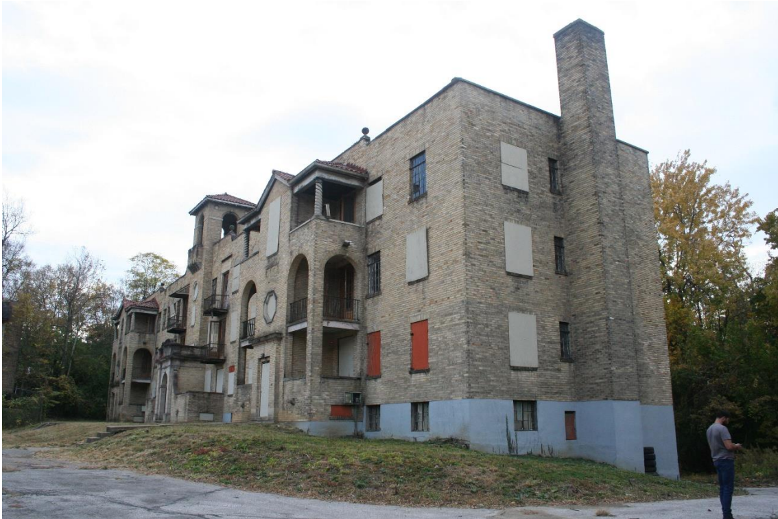
La Ventura, East (Front) and North (Side) Elevations
